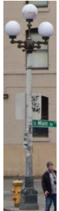
Street lighting example
