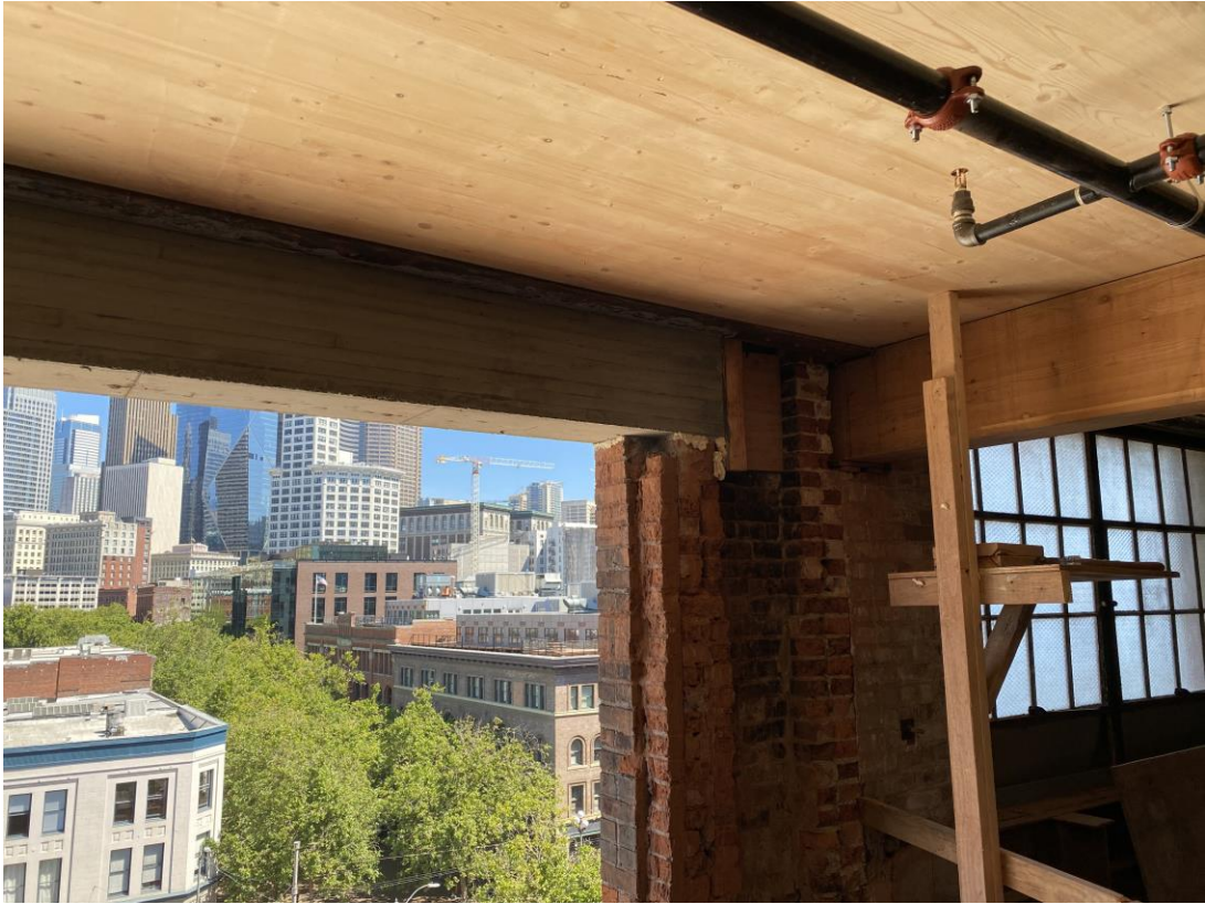
September 2021 – Support Work
