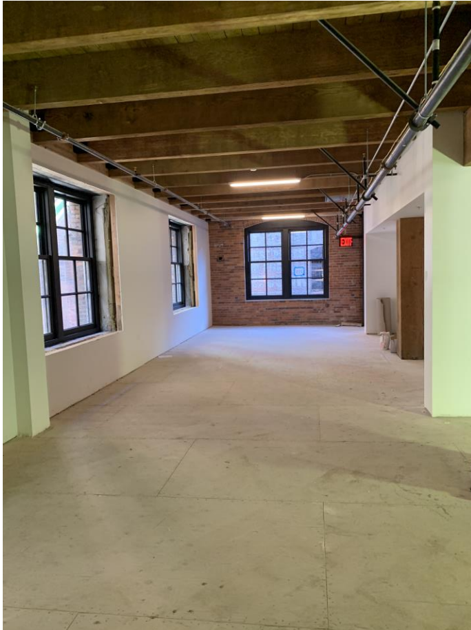
September 2021 – Office Shell
