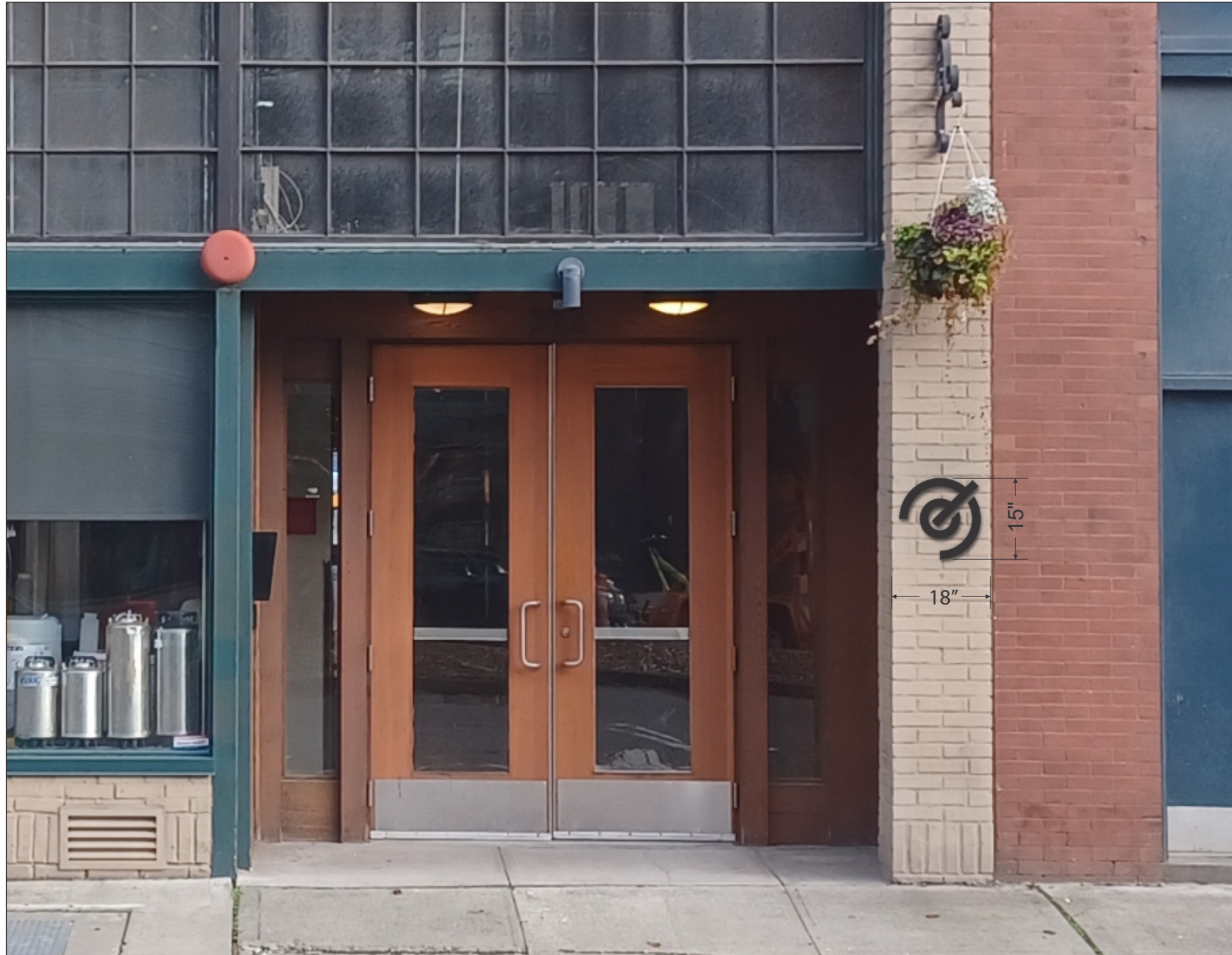
West Elevation - Non-Illuminated F.C.O Sign
