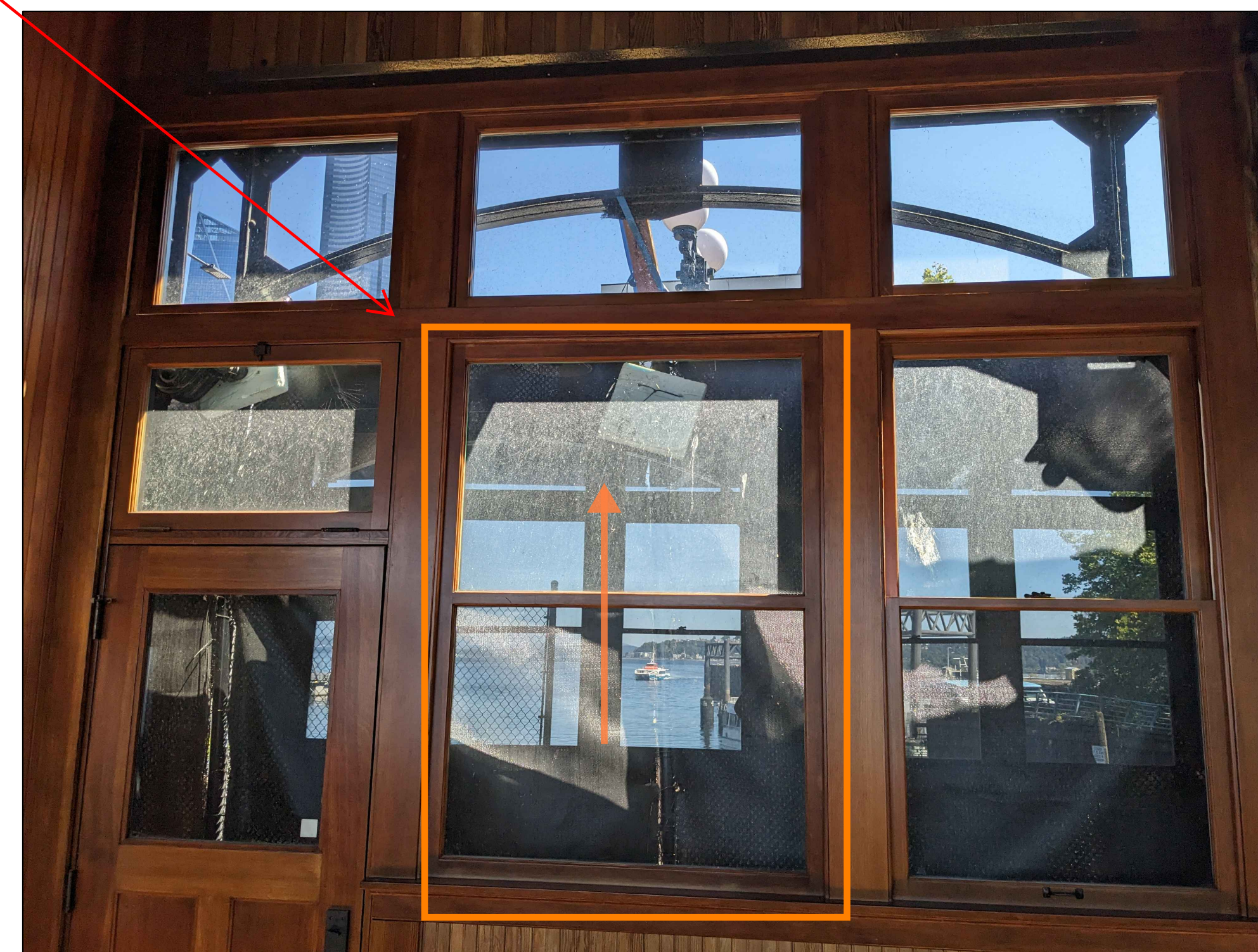
6 INTERIOR - WINDOW REPLACEMENT (typ) NTS
