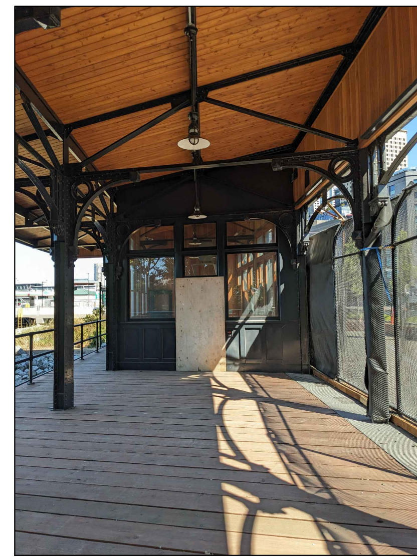
5 EXTERIOR - FACING NORTH NTS
