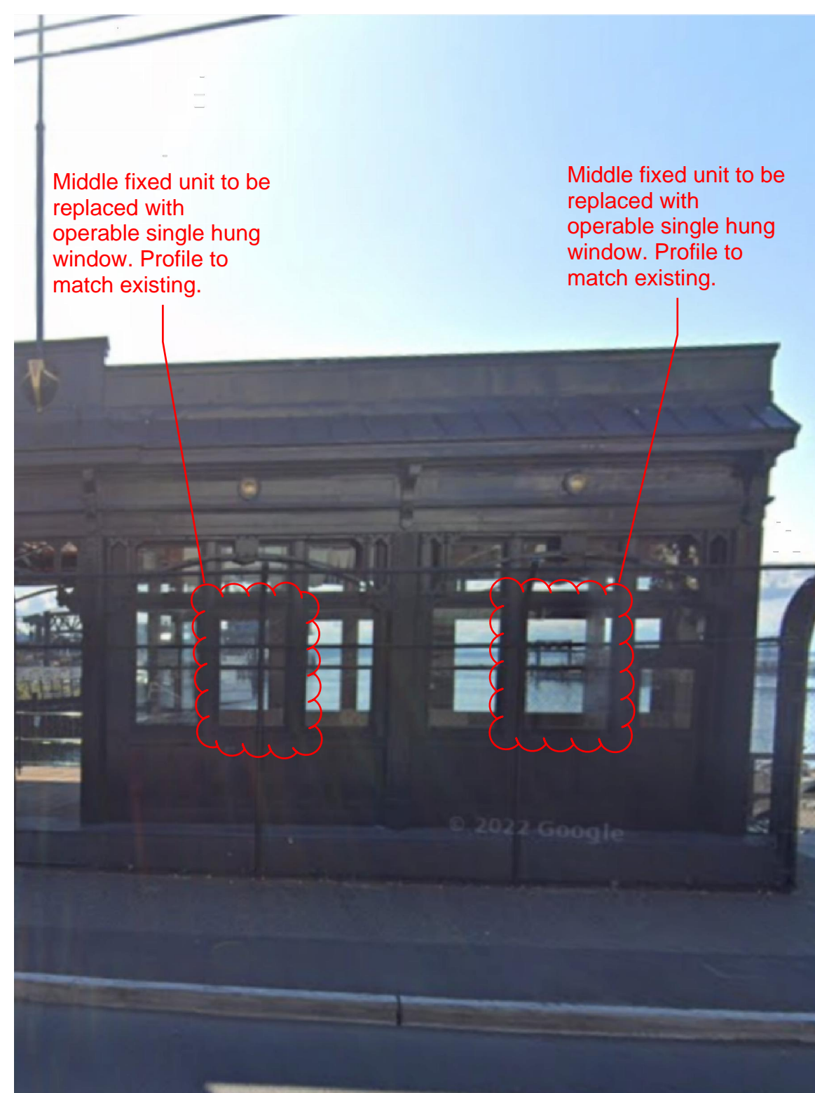
4 EXTERIOR ELEVATION EAST - WINDOW REPLACEMENT NTS
