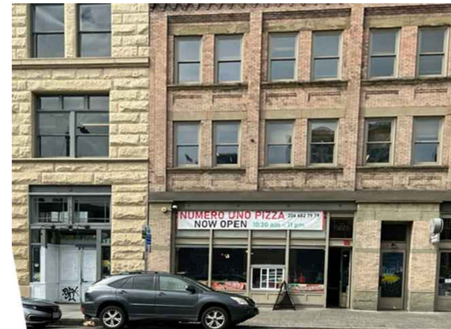
view from south, showing existing facade of spaces
