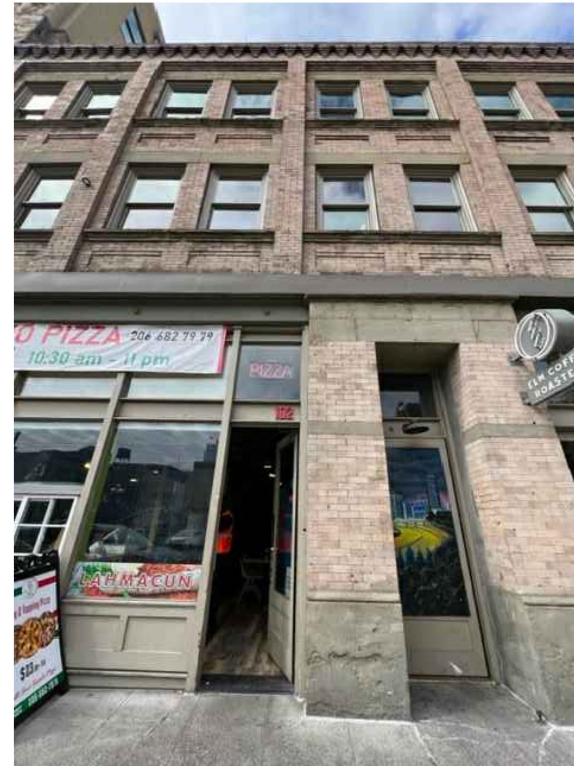
view from south, showing main entry as existing
