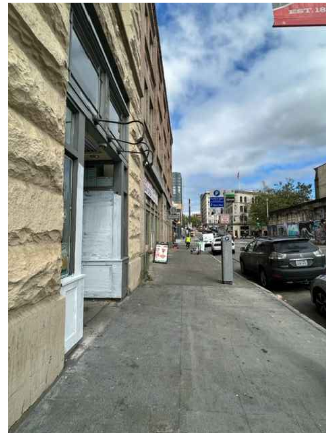
view from southwest, showing existing ground floor signage & entries
