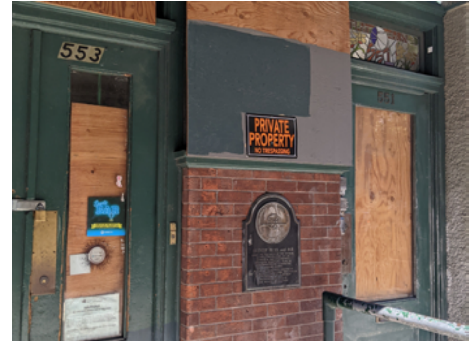
ENTRY TO PUB (LEFT) AND RESIDENCES (RIGHT) WITH STAINED GLASS TRANSOM
