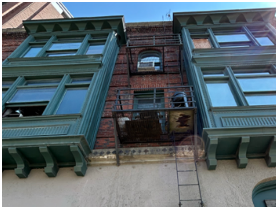
EXISTING FIRE ESCAPE
