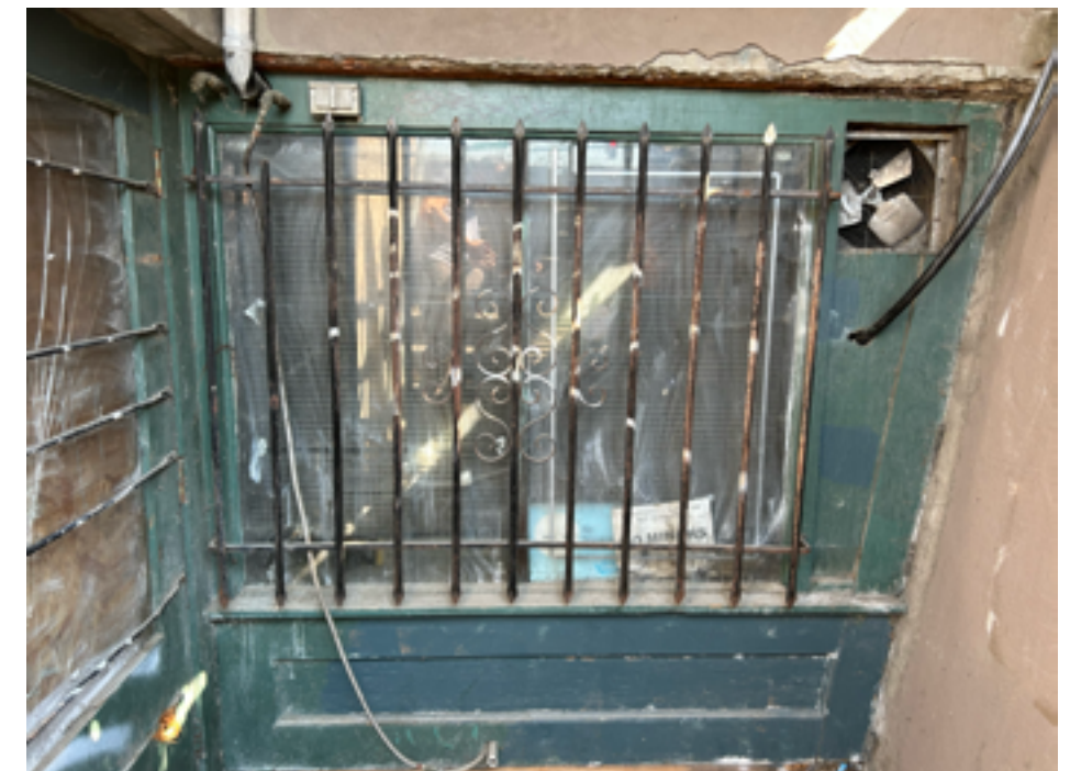
DOOR AND WINDOW WALL AT BOTTOM OF STEPS AT AREAWAY
