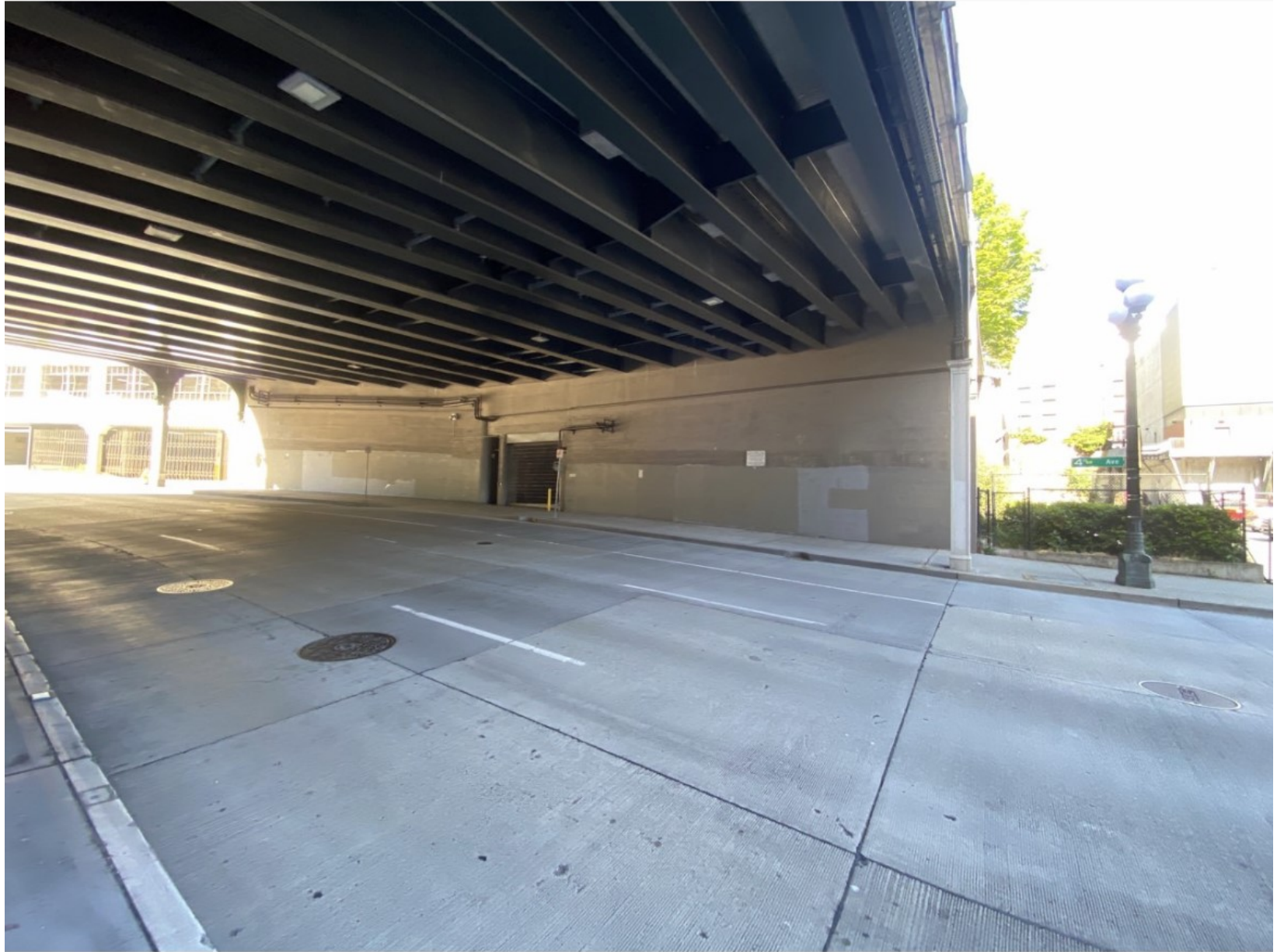
4th Ave Yesler Bridge embankment before mural
