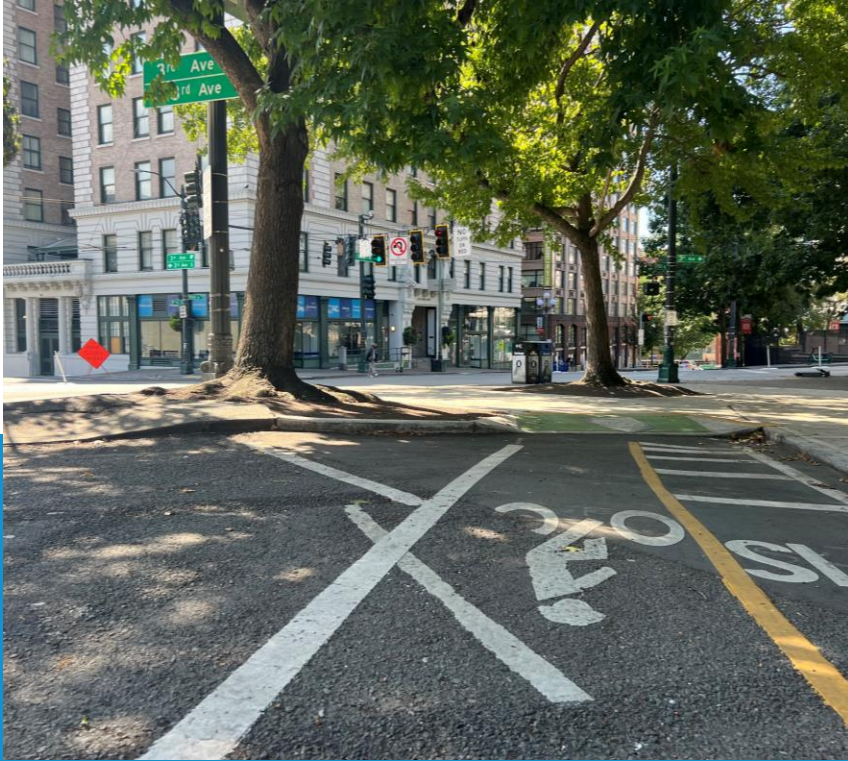
Looking west on Dilling Way toward 3 rd Ave
