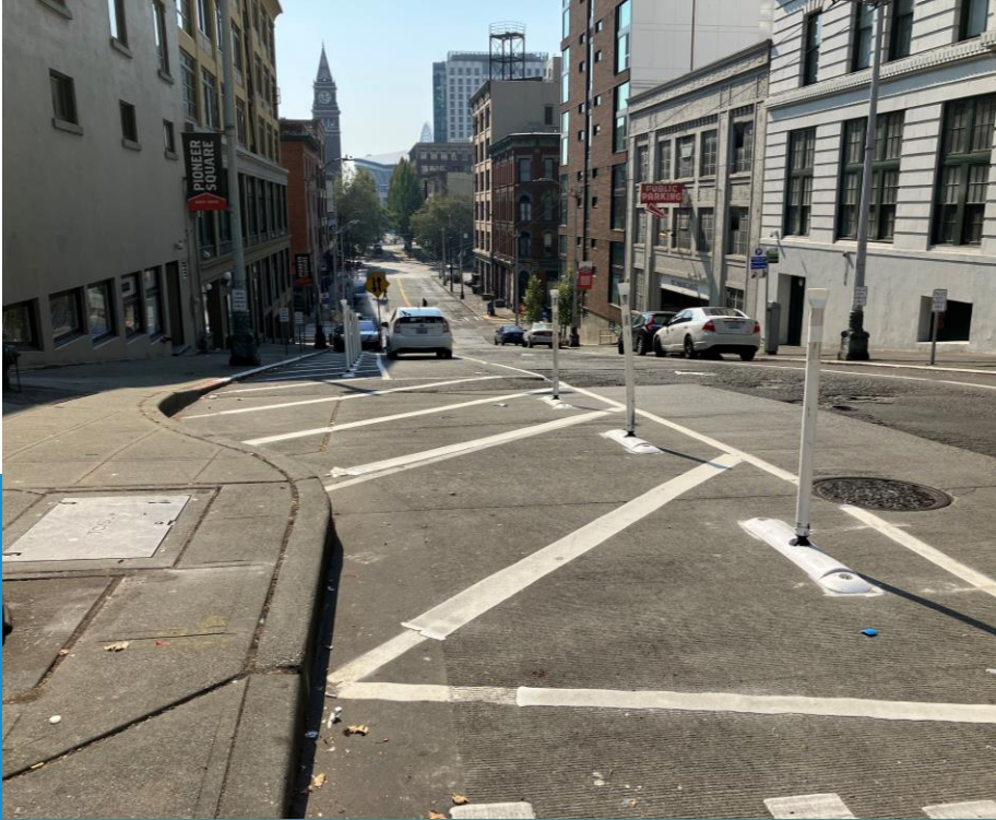
Looking south down 3 rd Ave
