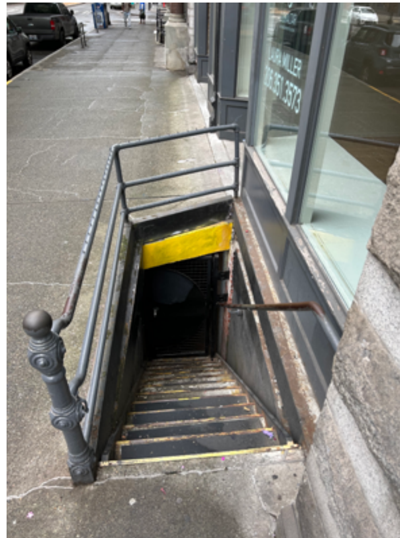
PICTURE FROM TOP OF STAIR (NORTH)
