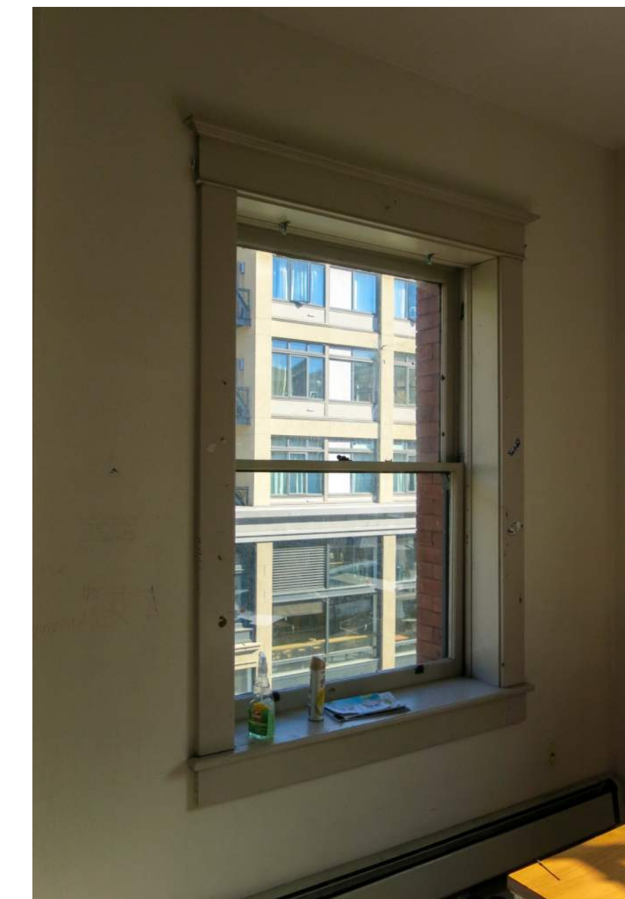
UNIT 411 WINDOW INTERIOR 2021
