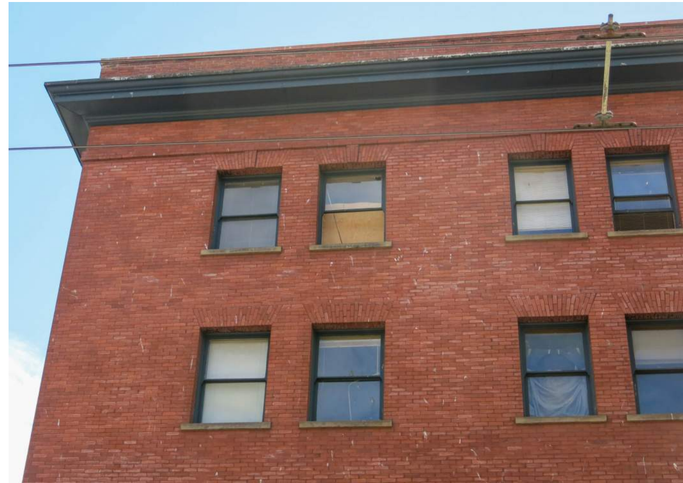
NORTH ELEVATION UPPER WINDOWS 2021
