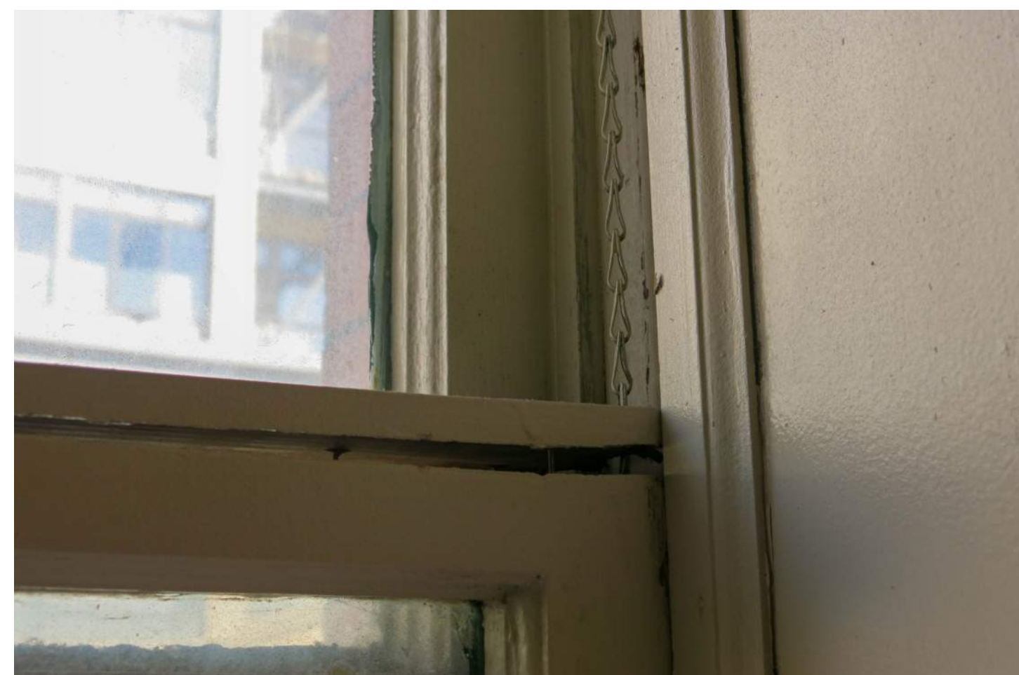
UNIT 215 WINDOW INTERIOR 2021
