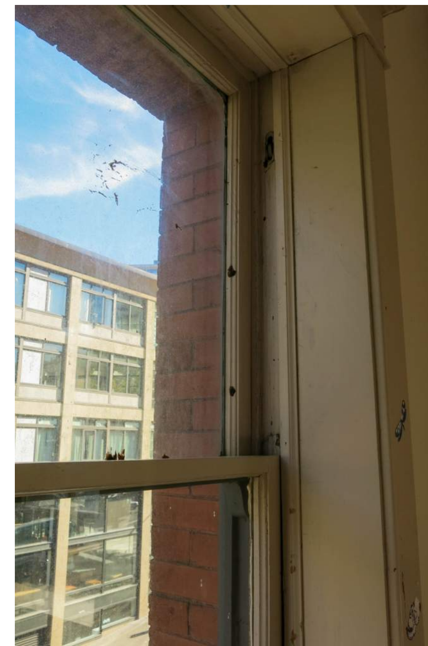
UNIT 411 WINDOW INTERIOR 2021
