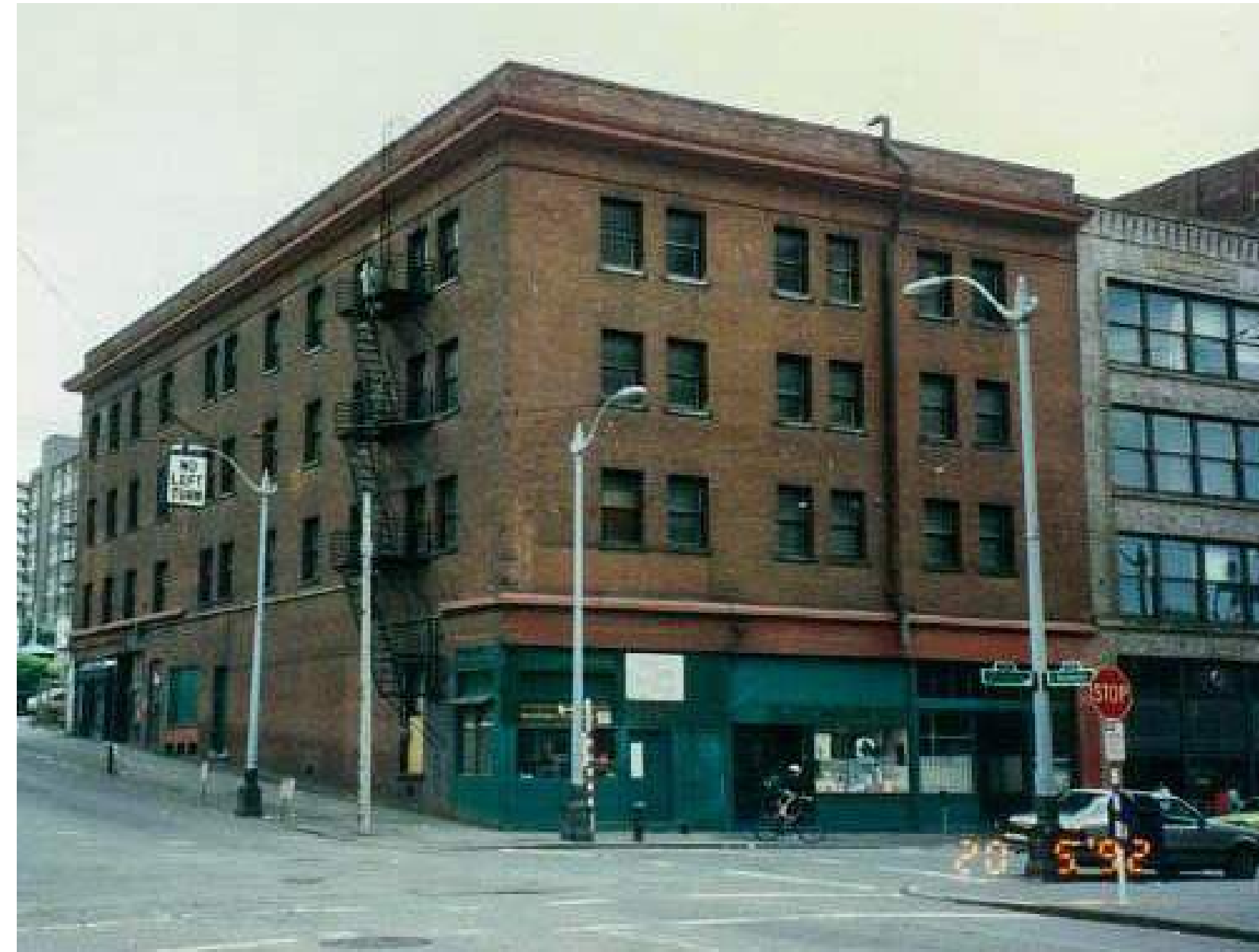
NORTHWEST ELEVATION PRIOR TO RENOVATION 1992
