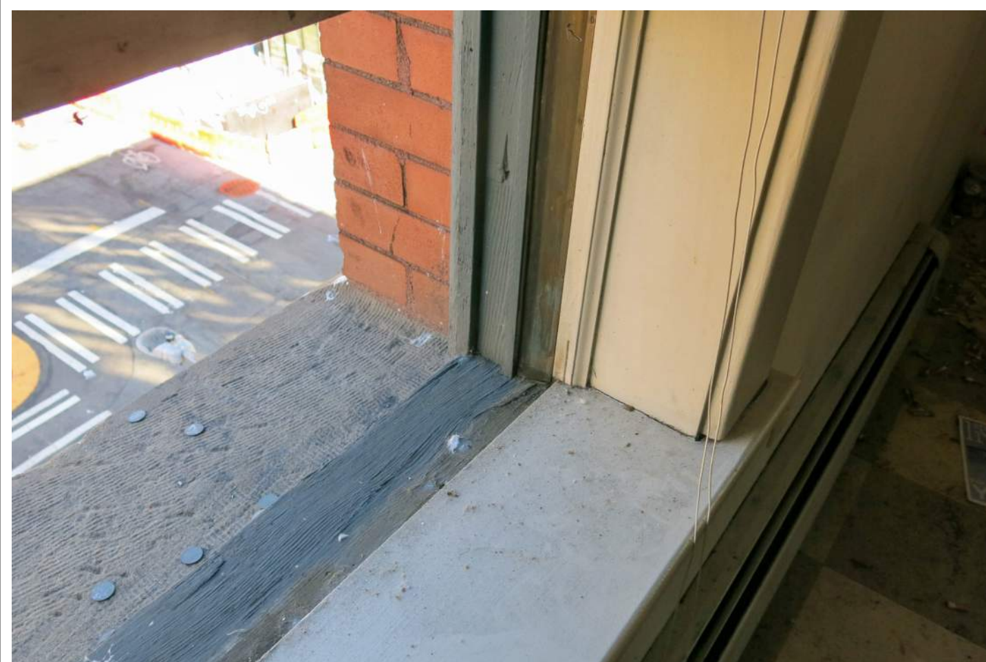
UNIT 401 WINDOW INTERIOR 2021
