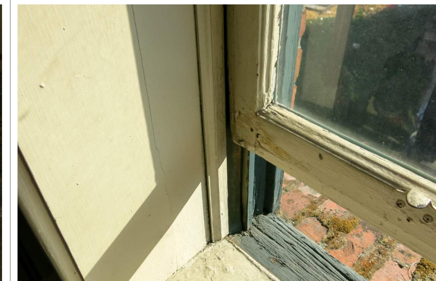
UNIT 407 WINDOW INTERIOR 2021
