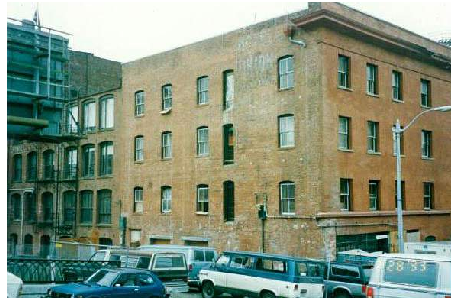
EAST/NORTH ELEVATIONS DURING RENOVATION 1993
