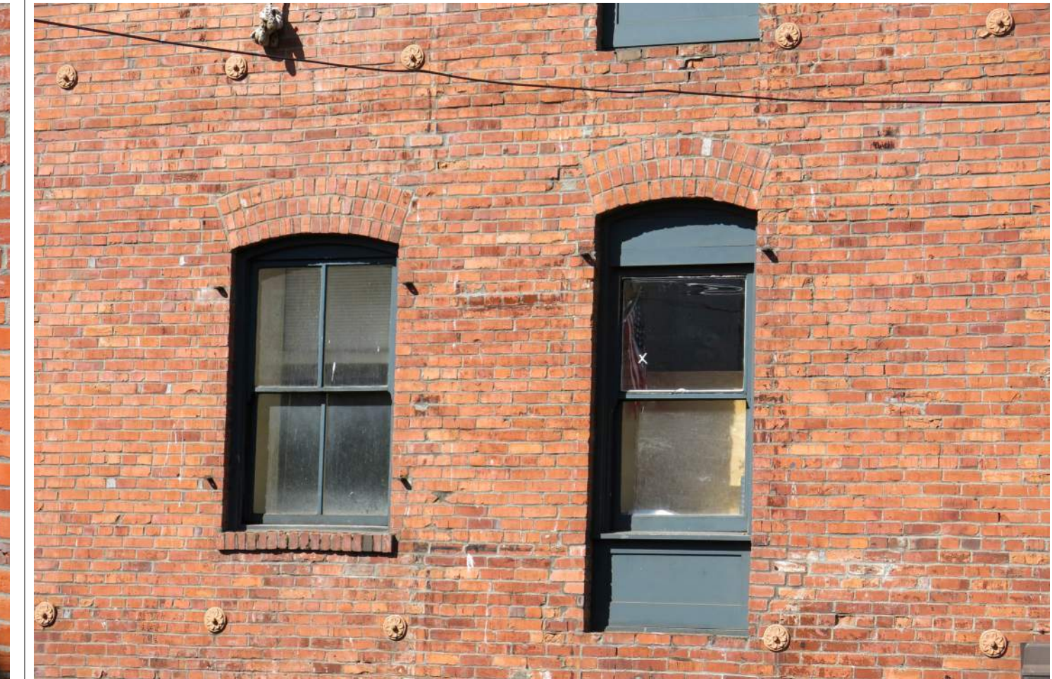
EAST ELEVATION UPPER WINDOWS 2021
