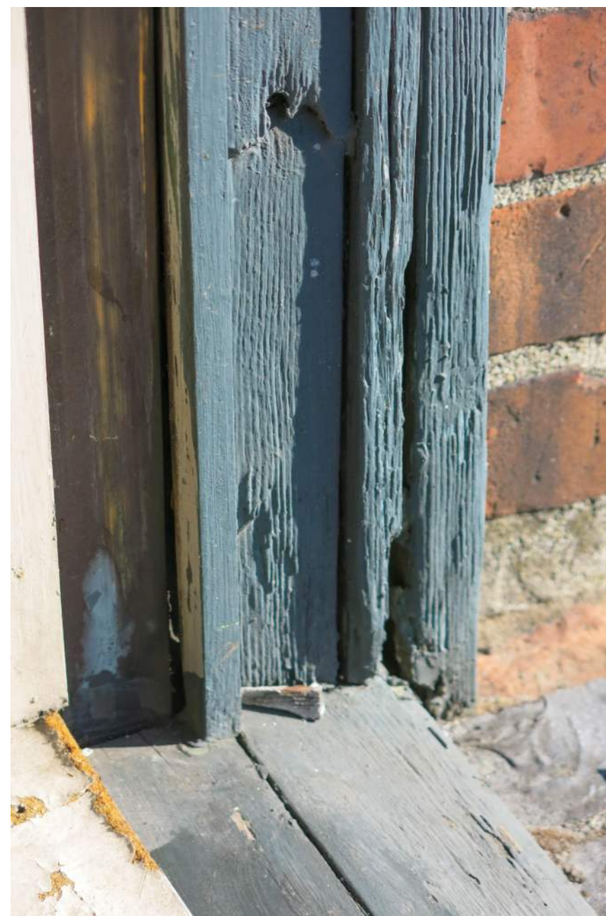
UNIT 411 WINDOW INTERIOR 2021
