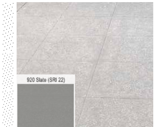
Sidewalk concrete paving and roadway concrete panels (travel lane) to be light grey meeting PSPB guidelines for lamp black in cement concrete mix. 2'x2' scoring.
