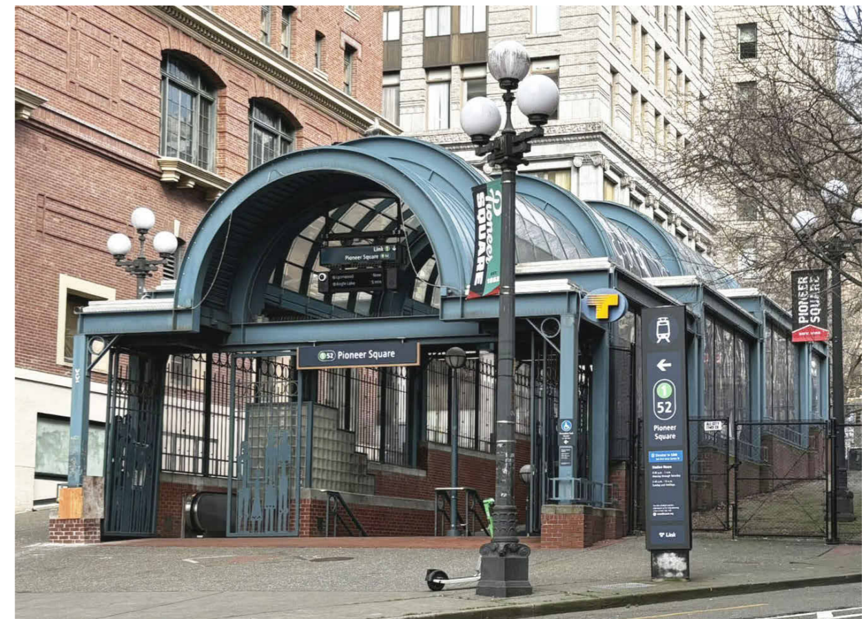
PREFONTAINE HEADHOUSE - 2ND AVE ENTRY
