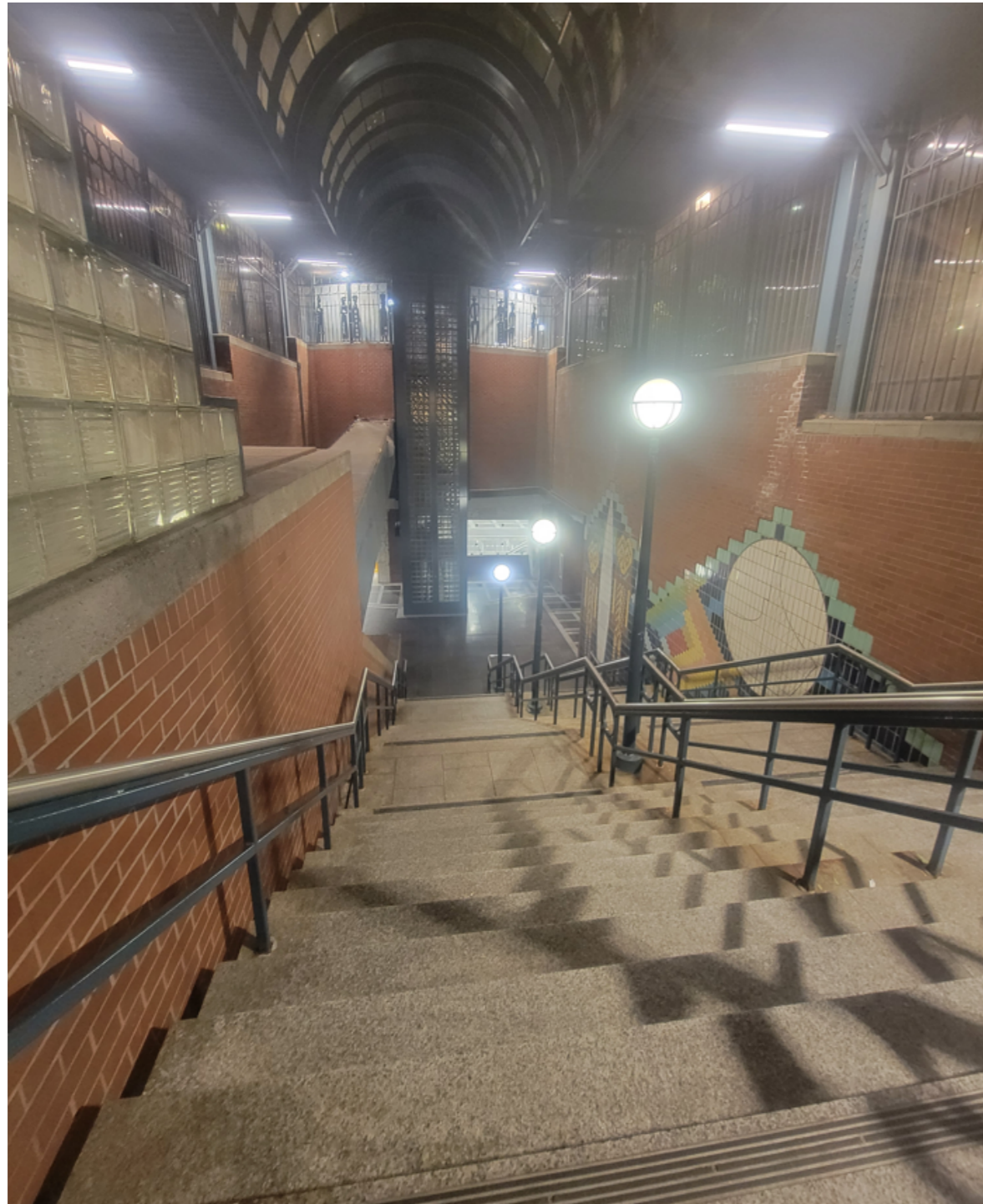
Pioneer Square Station (Prefontaine) at the stair areas
