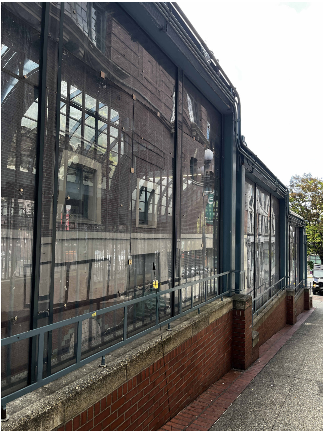
EXISTING FACADE - WEST
