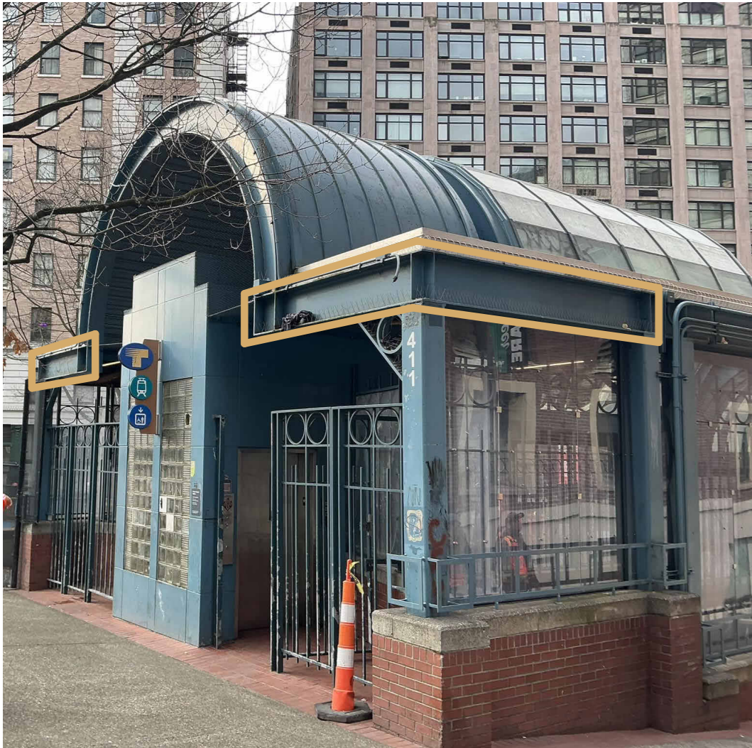
EXISTING FACADE - 3RD AVE / ELEV ENTRY
