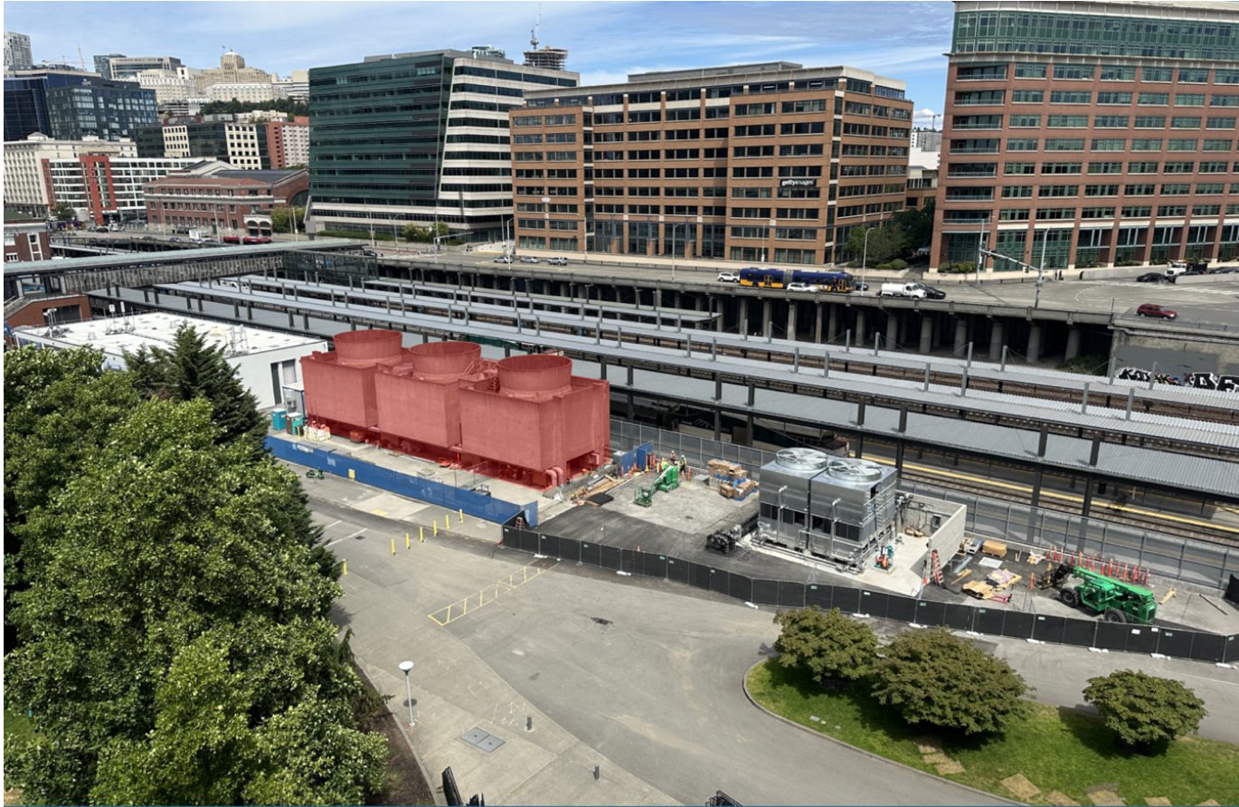
Current overview from right to left: 1. New Fluid Cooling Towers per DONH-COA-01552; 2. Decommissioned Towers to be demolished per DONH-COA-01553 and the proposed site for the EL5B; 3. Existing Annex.
