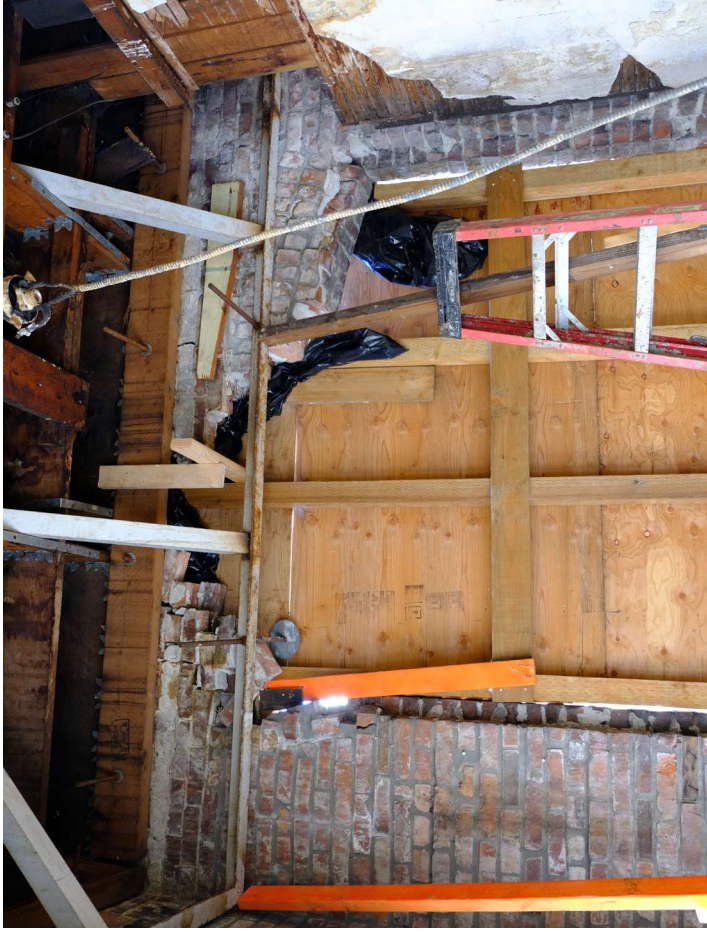
collapsing load-bearing brick wall at window in north wall of 2nd story of south annex
