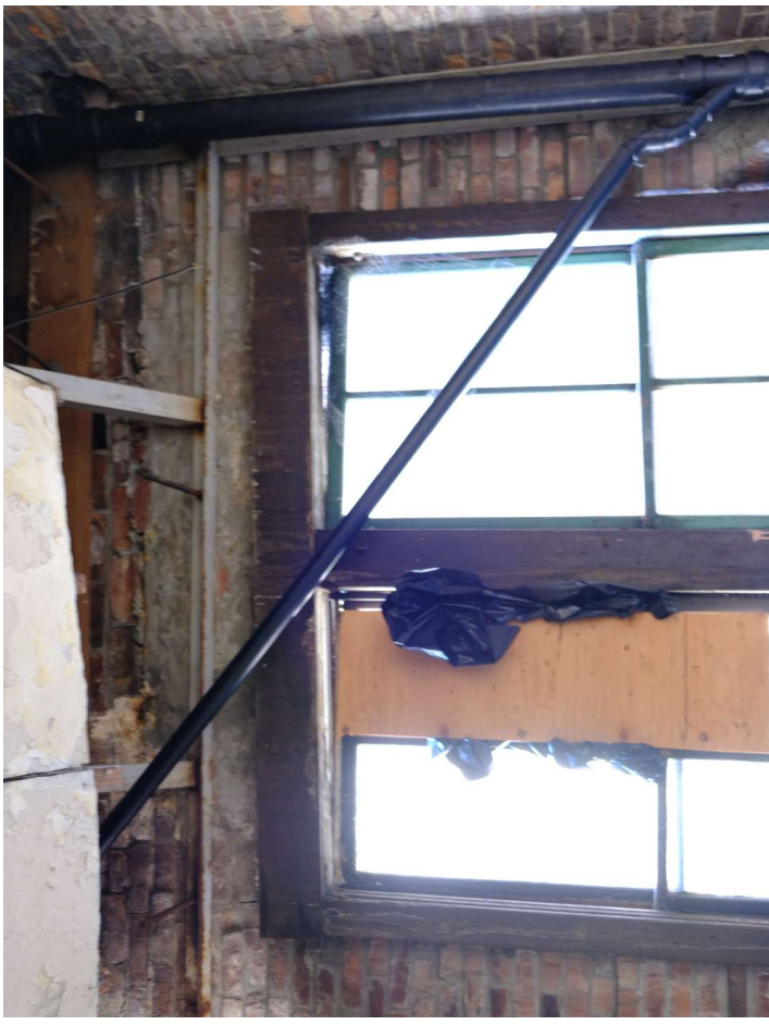
failing lintel at 2nd story window in south annex
