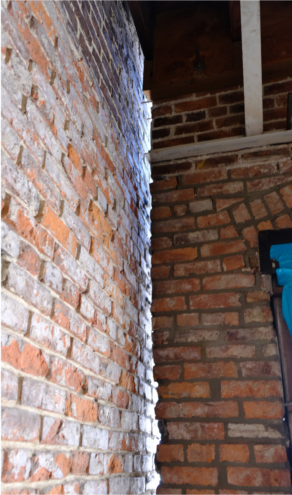
3" daylight gap between west wall of south annex and neighboring building to the south.
