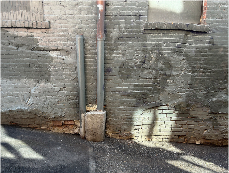
deformation of load-bearing brick at west wall of north annex
