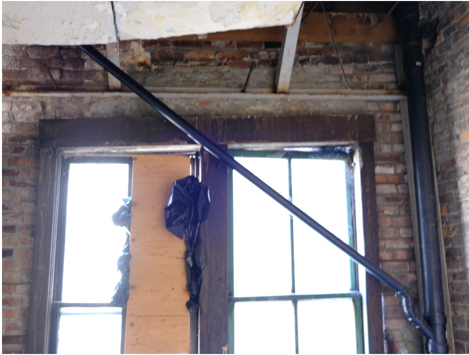
failing lintel at 2nd story window in south annex
