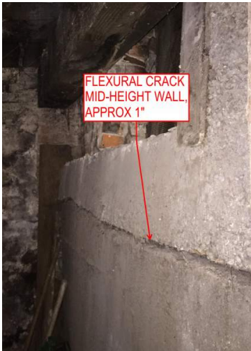
Figure 4: Basement Wall Flexural Failure
