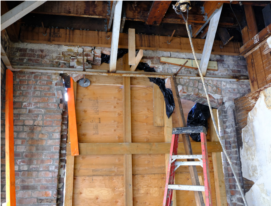
collapsing load-bearing brick wall at window in north wall of 2nd story of south annex
