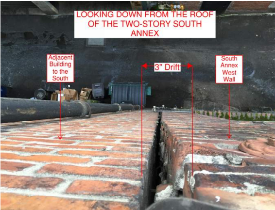
Figure 1: Northerly Drift- South End of Building
