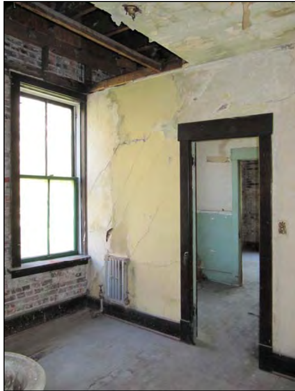
Figure 63. Bottom right, detail of a corner guestroom where plaster has been removed from walls, and the ceiling removed to access framing.
