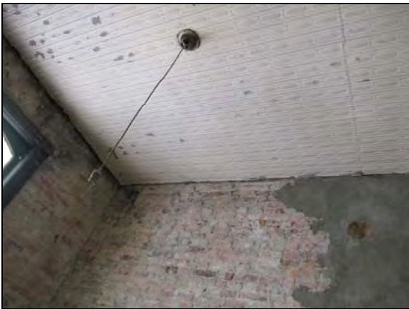
Figure 63. Bottom right, detail of a corner guestroom where plaster has been removed from walls, and the ceiling removed to access framing.
