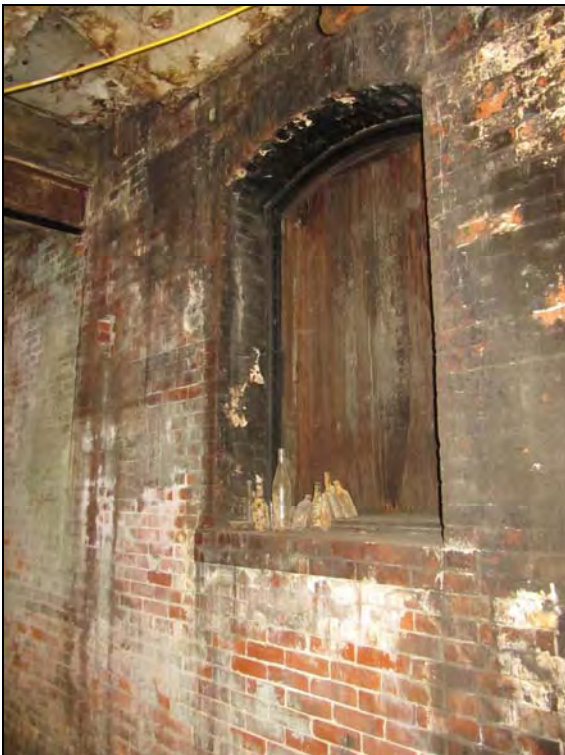
Figure 42. Below, infilled arched head opening between the basement and areaway.
