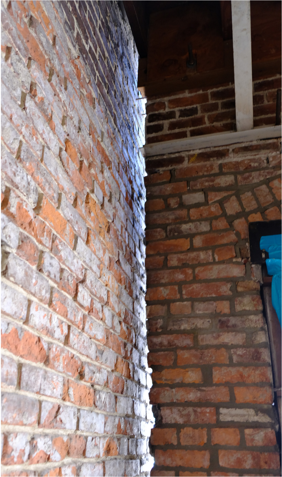
3" daylight gap between west wall of south annex and neighboring building to the south.
