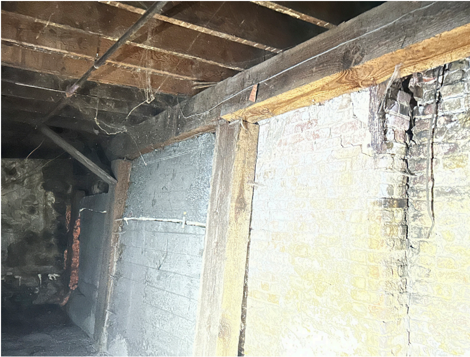
west wall of north annex at basement level is leaning away from building
