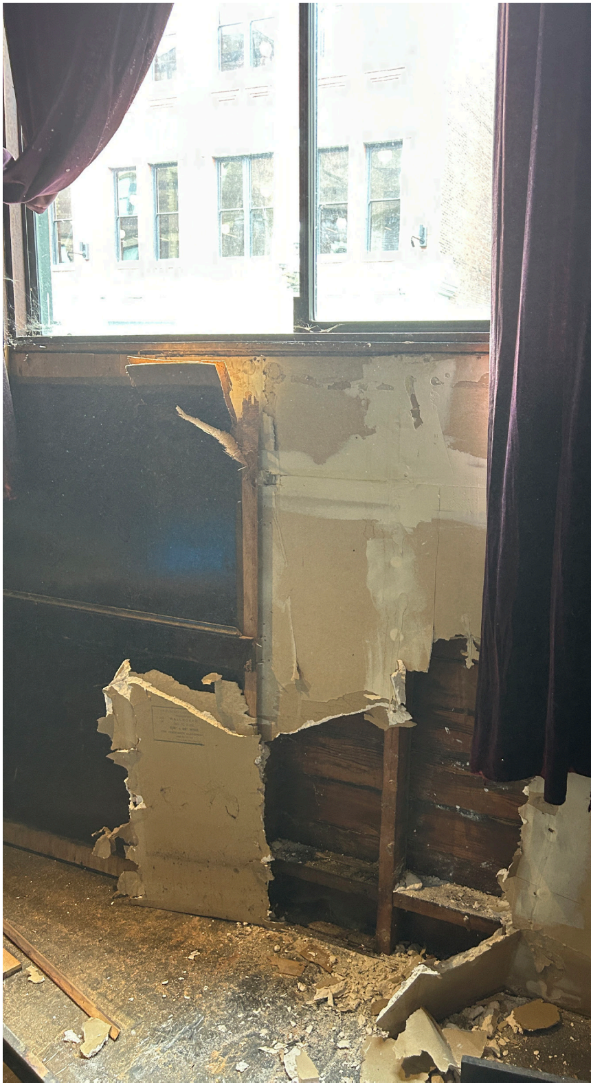
demolition of wall shows assembly of gwb, 2x4's and horizontal wood siding
