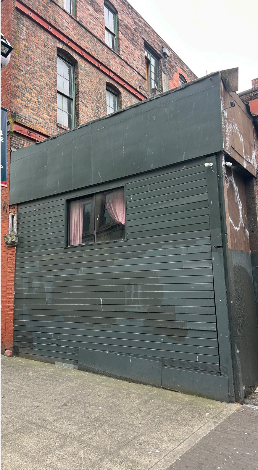
horizontal wood siding at annex, seen from exterior
