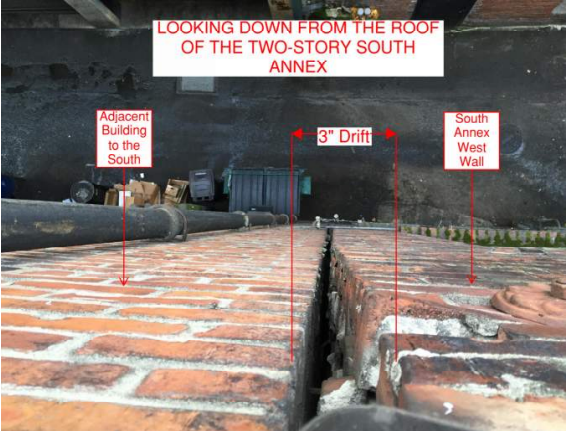
Figure 1: Northerly Drift- South End of Building
