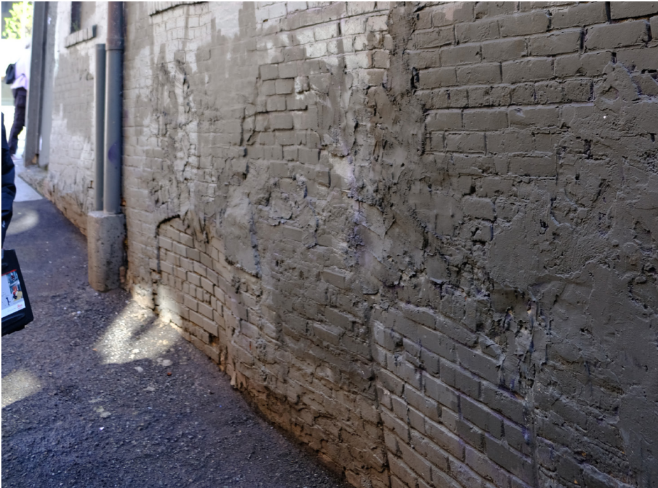
deformation of load-bearing west wall of north annex along the alley
