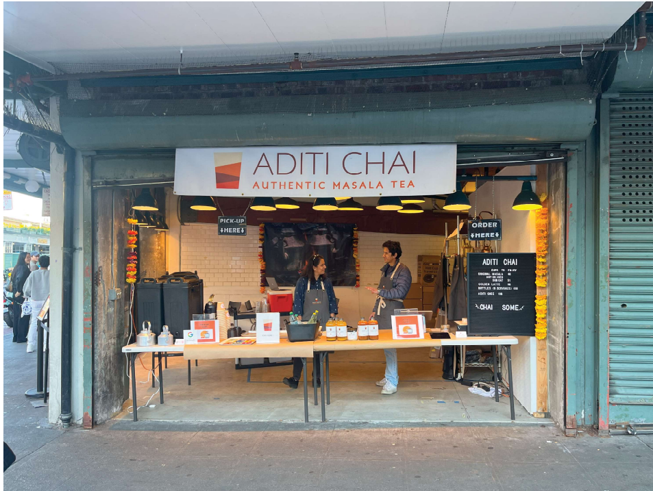
Existing South Storefront
