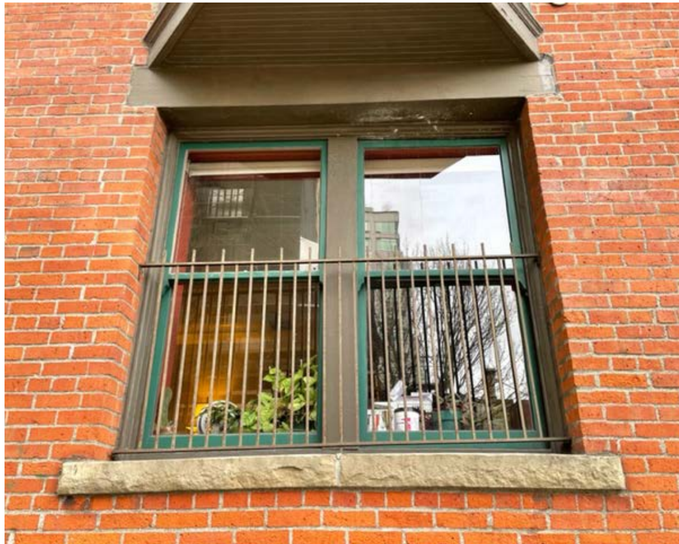
EXTERIOR WINDOW PHOTO TAKEN FROM VIRGINIA ST FACING EAST
