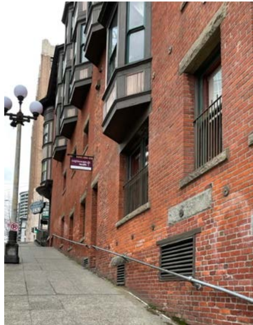
EXTERIOR AT VIRGINIA ST PHOTO TAKEN FROM VIRGINIA ST FACING NE
