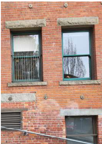
WINDOW GUARD CENTRAL WINDOWS
