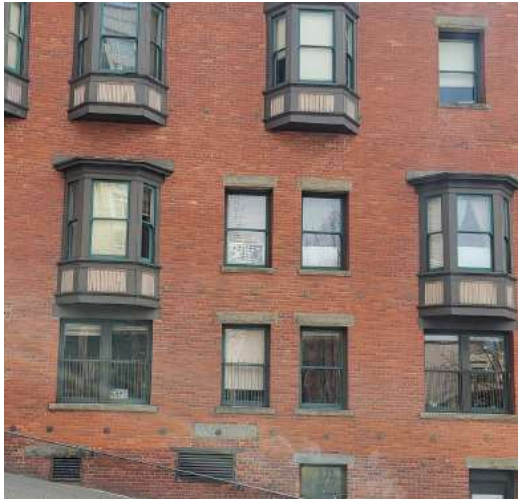
EXISTING WINDOW GUARDS ON NW FACADE
