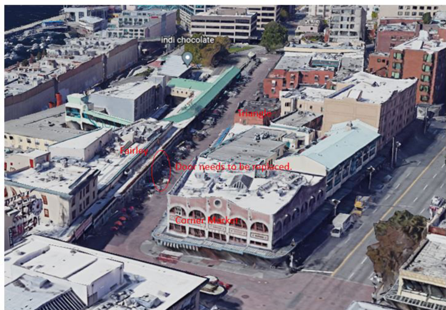
Attachment 5: Adjacent street and buildings
