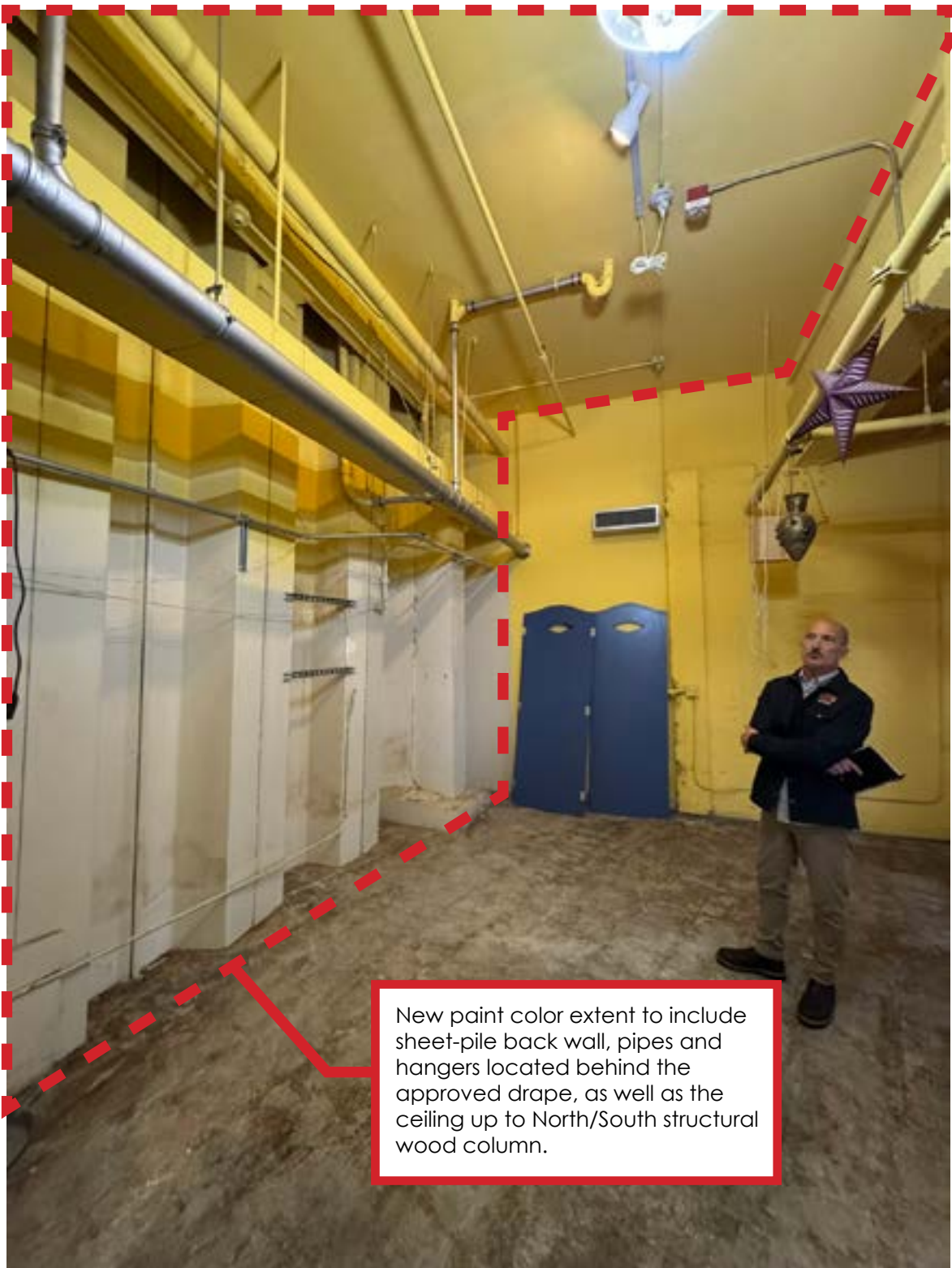
Existing Conditions - Looking South
