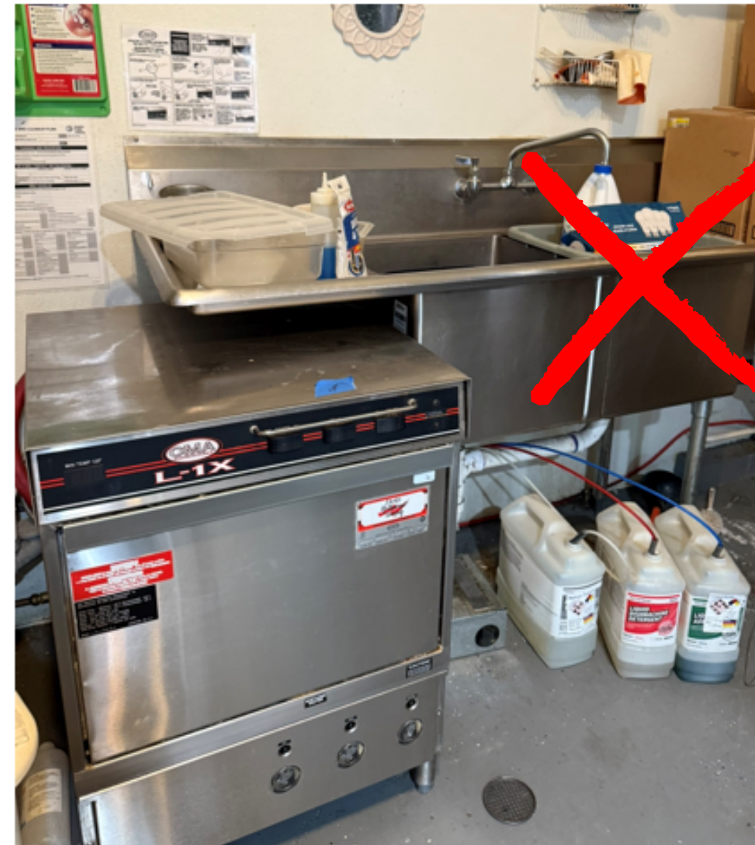
Existing east wall replacing 2-compartment sink with 3-compartment sink. Dishwasher remains - BOH
