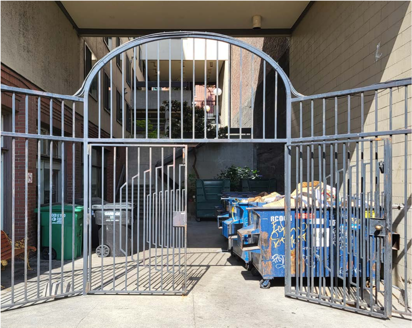
PRECEDENT AT PIKE PLACE MARKET PHOTO TAKEN FROM POST ALLEY FACING NORTHWEST
