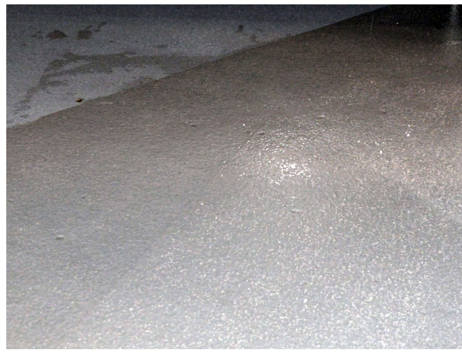
PRODUCTION FLOOR - EPOXY 15
