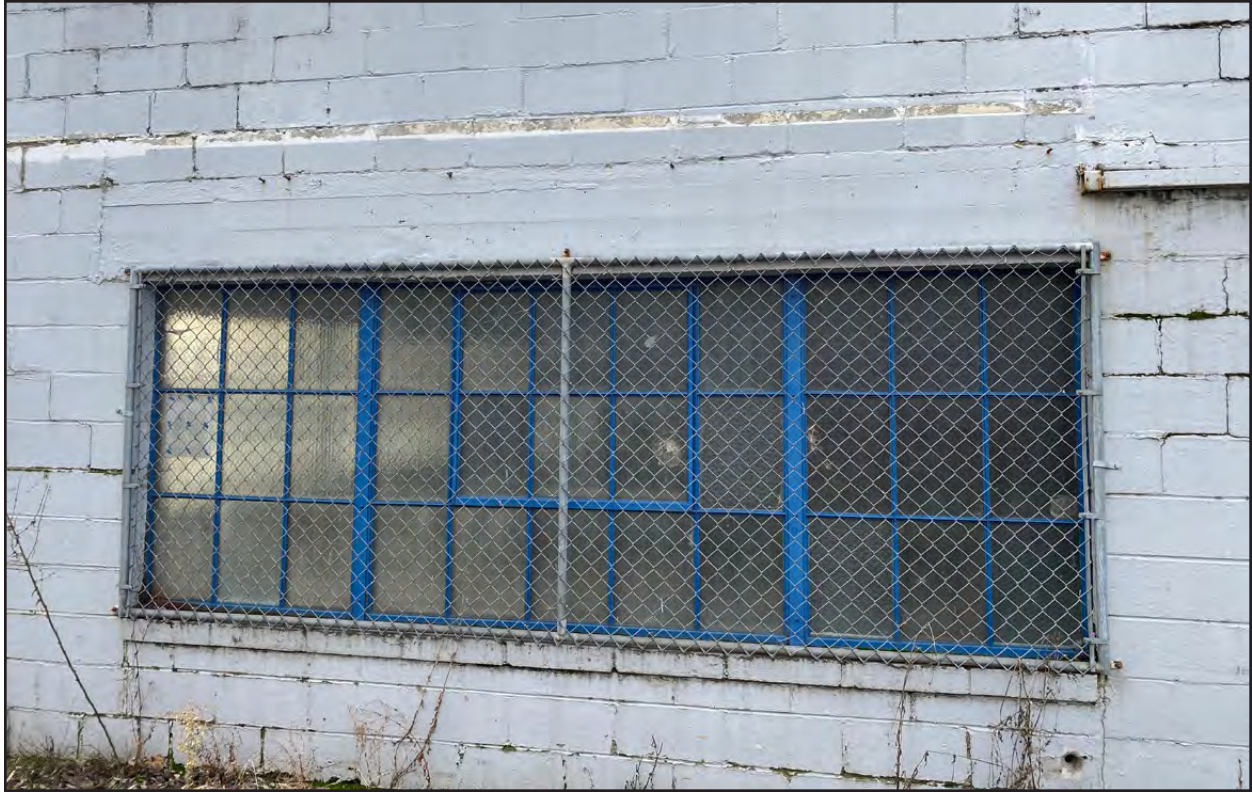
Figure 13 • 1265 S King Street, detail of industrial steel-sash window at the eastern façade
