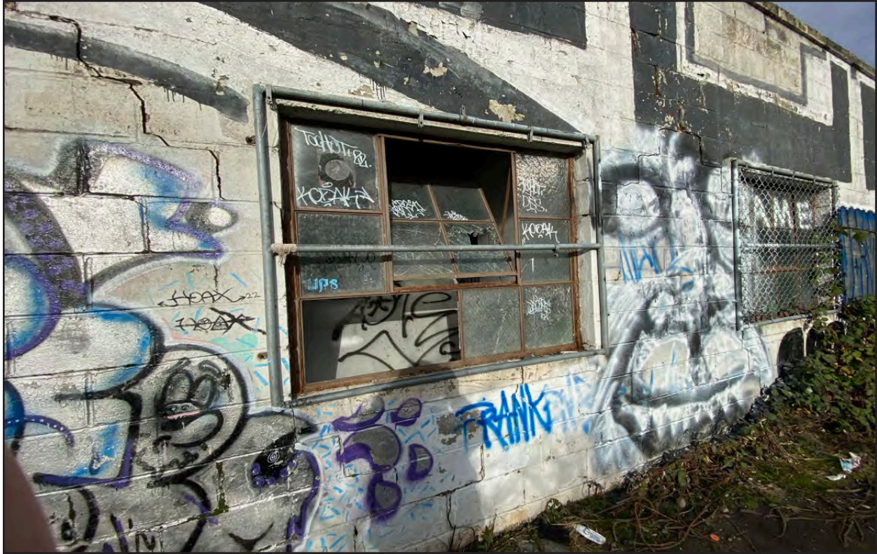
Figure 17 • 1265 S King Street, detail of industrial steel-sash window at southern façade
