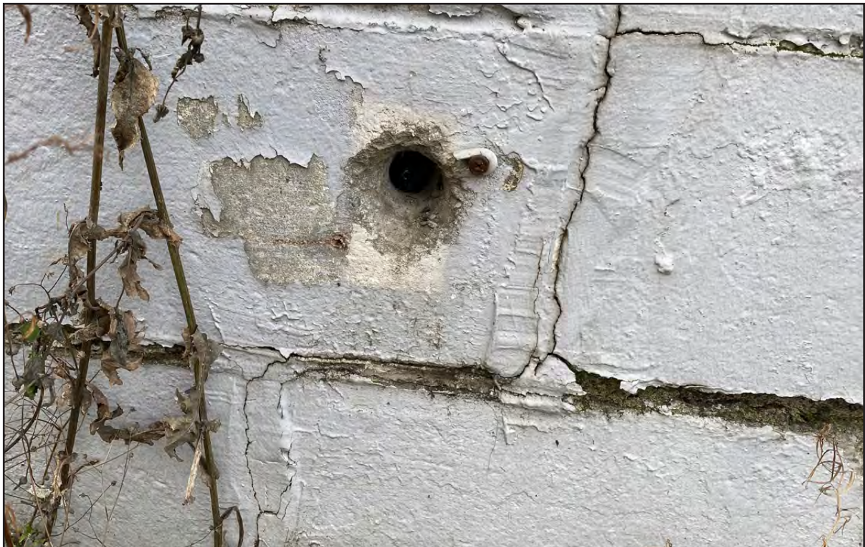
Figure 14 • 1265 S King Street, detail of hollow CMU and CMU condition
