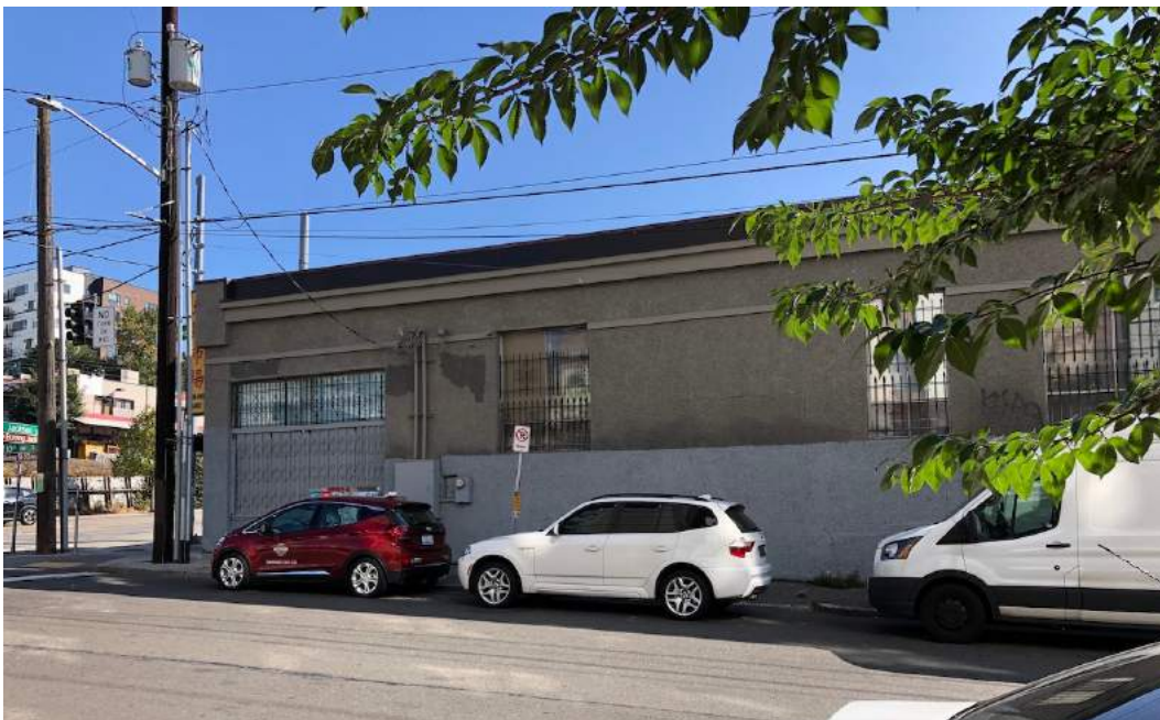
View northeast from 10th Ave S., showing the northern portion of the west façade (1001 S. Jackson).
