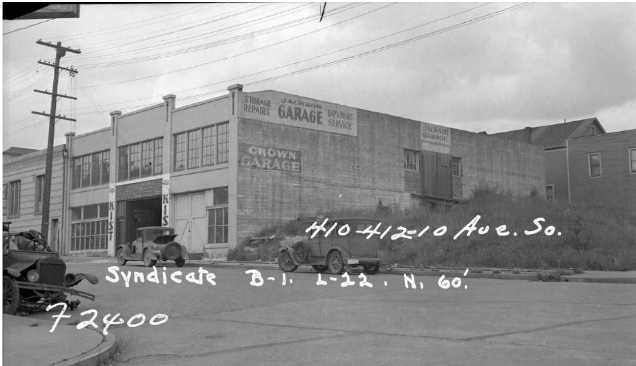
Two views in 1937. Top view is looking southeast at the north and west façades of 1001 S. Jackson; bottom view is looking northeast toward the west and south façades of 410 10th Ave S. (King County Tax Assessor property record, Puget Sound Regional Archives)
