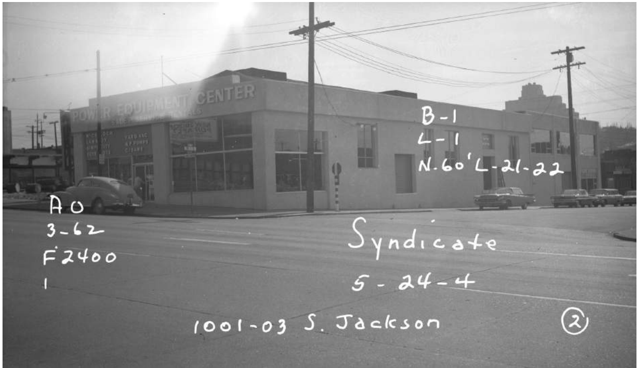
A 1962 view looking southeast at the north and west façades of 1001 S. Jackson and the west façade of 410 10th Ave S., following building alterations. At this point the buildings were consolidated as one tax parcel and “unified” visually by a single architectural treatment. (King County Tax Assessor property record, Puget Sound Regional Archives)
