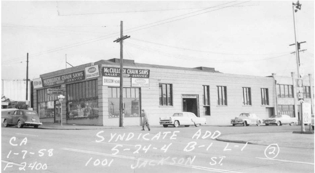
A 1958 view looking southeast at the north and west façades of 1001 S. Jackson, following building alterations. Note the storefront has been pulled flush to the sidewalk and the west windows have been changed. (King County Tax Assessor property record, Puget Sound Regional Archives)
