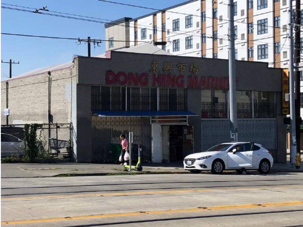
View southwest toward the building's primary north façade (1001 S. Jackson).
