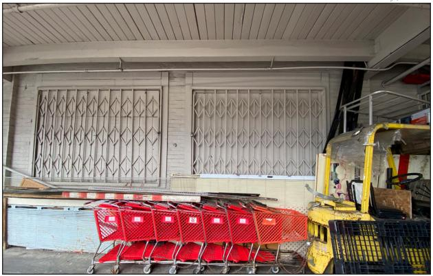
Figure 14 • Non-original boarded up opeinigns at loading dock, building 1
