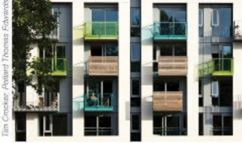
Use of balconies to provide depth, color and interest to building facade
