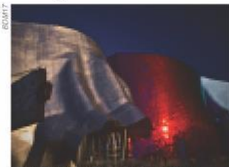
Glare caused by reflective surface of building
