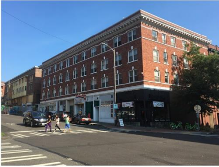
Contributing building with an example of projecting cornice
