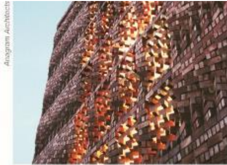
Bricks used for facade articulation
