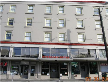
Example of transoms and large bays
