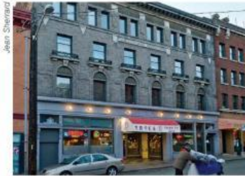
Typical facade articulation in Chinatown
