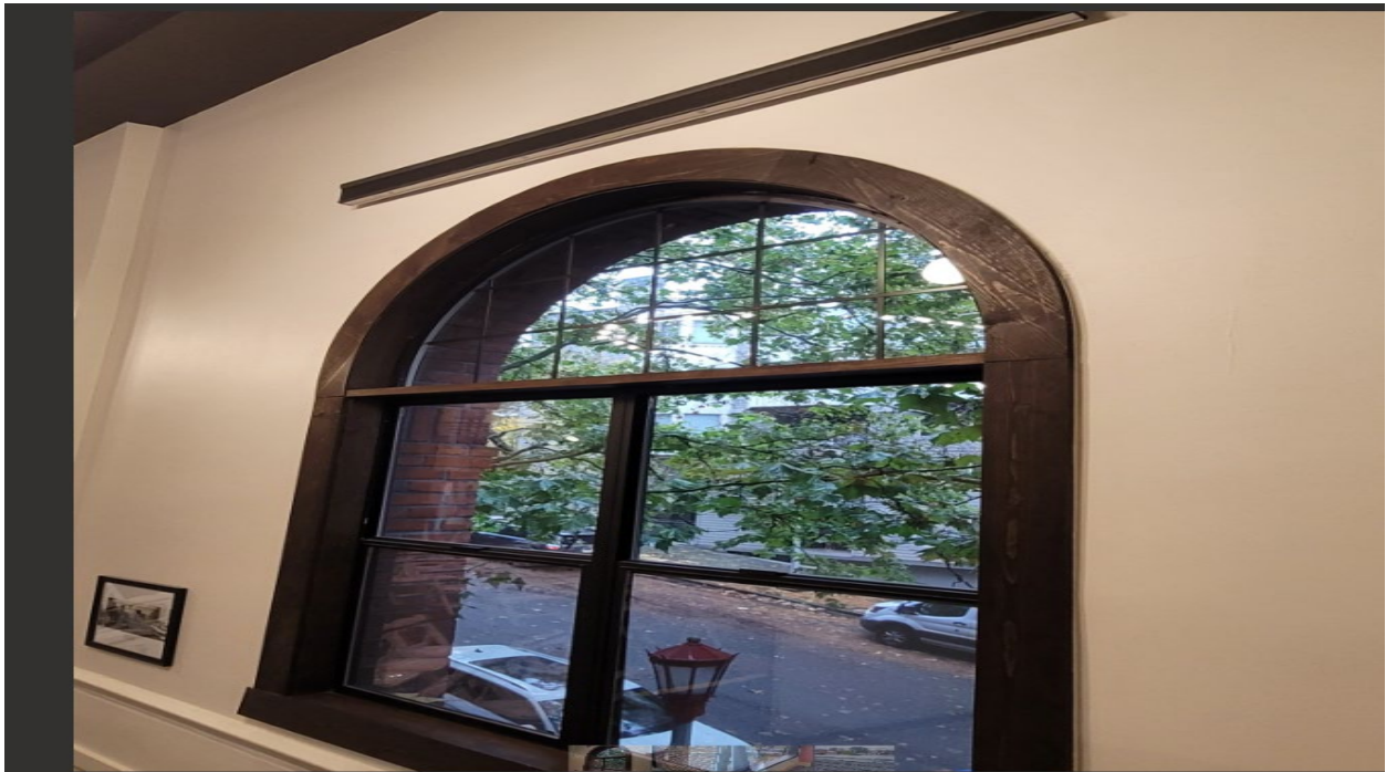
10. Motorized window shade example, in theatre.
