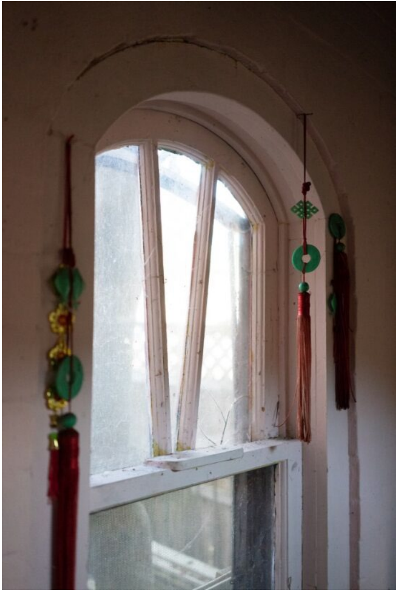
Interior details, pre-rehabilitation, 2023
