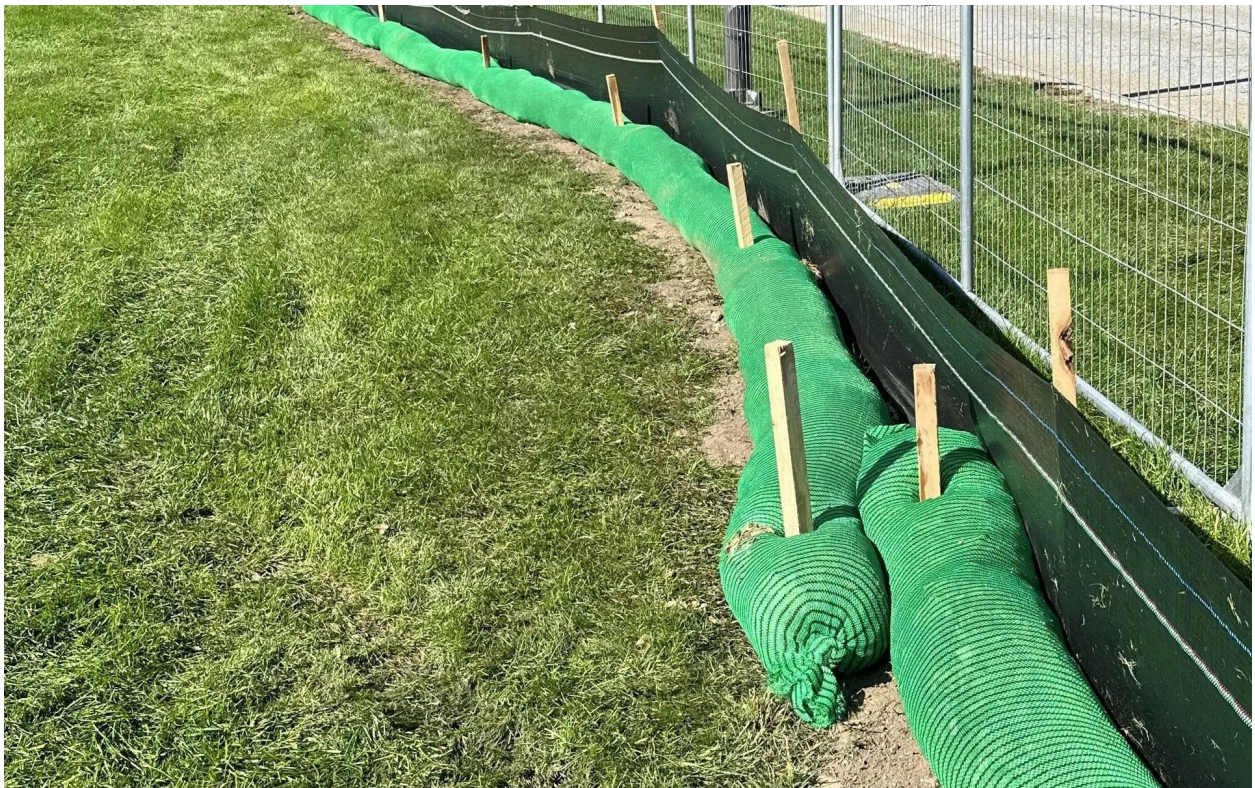
Example of compost sock and silt fence, used as necessary.
