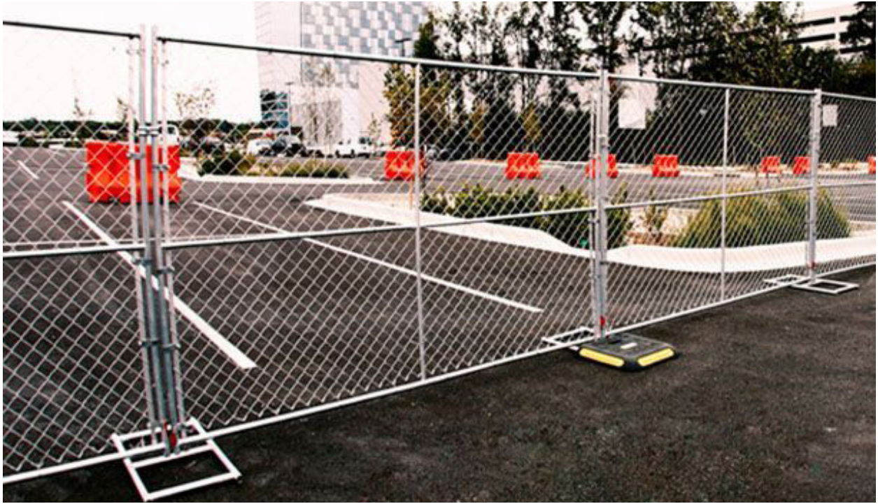
Example of temporary construction fencing. Aluminum chain-link finish.
