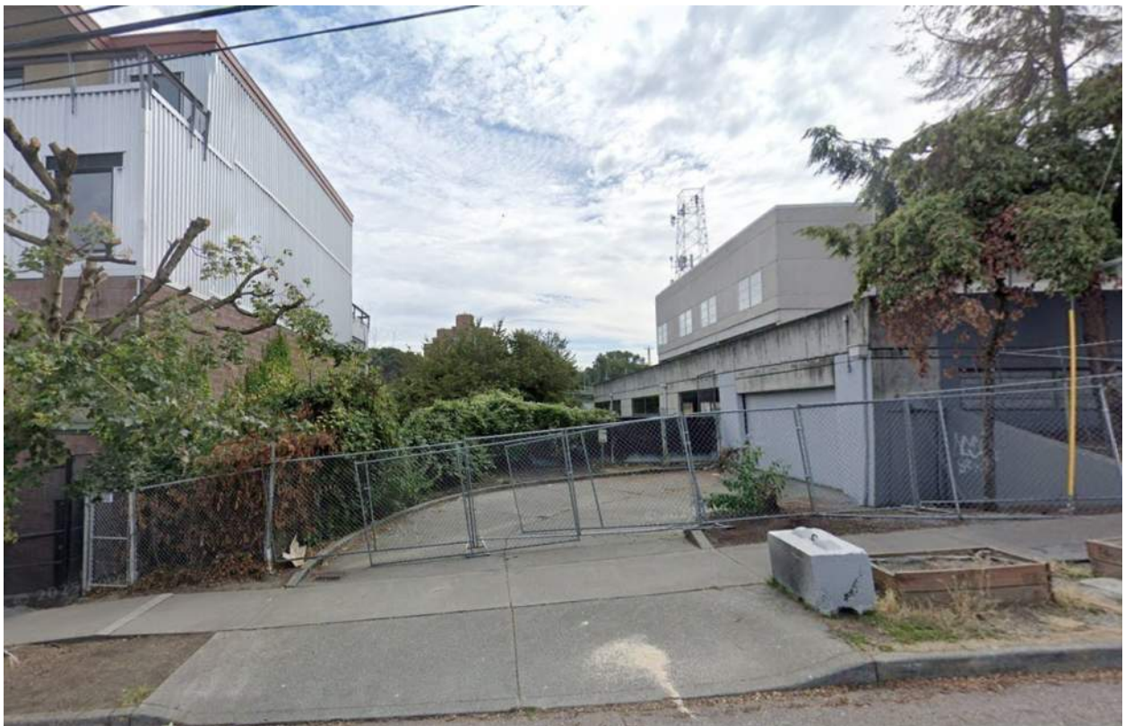
View on S Weller St along East Property Line
