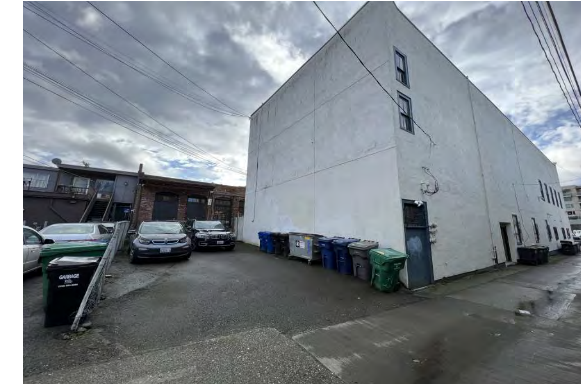
E ALLEY ROW, LOOKING SOUTH AT EMPLOYEE PARKING LOT, ADJACENT PARCEL TO ARK LODGE CINEMAS
