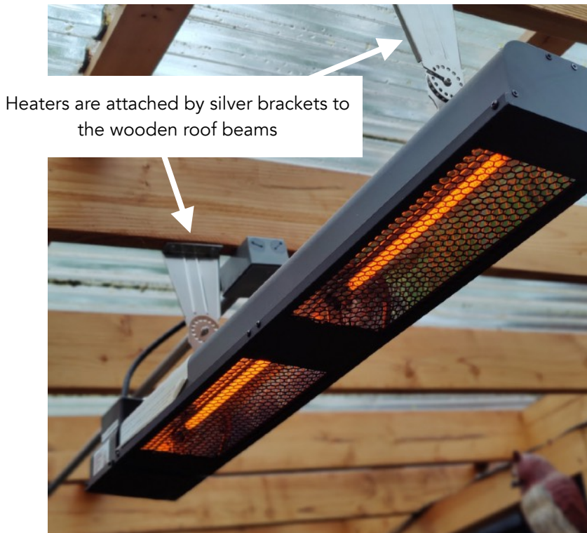
Photo 41: heater attachment detail
