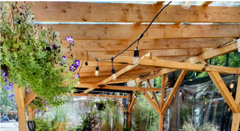
Photo 9: Detail of Douglas Fir structure with lighting and flower planters
