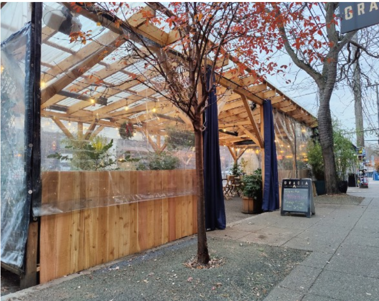
Photo 16: Patio shown from the sidewalk looking southward. This railing is constructed of weather-treated, cane-detectable Douglas Fir and Cedar planks.
