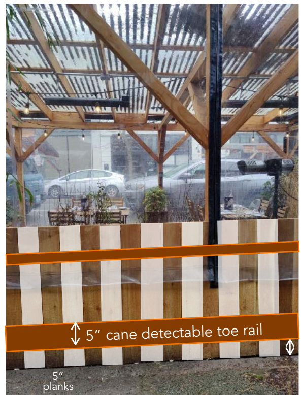
Photo 17: A 5" wide horizontal toe rail will also be added, measuring 2" from the sidewalk as pictured.
