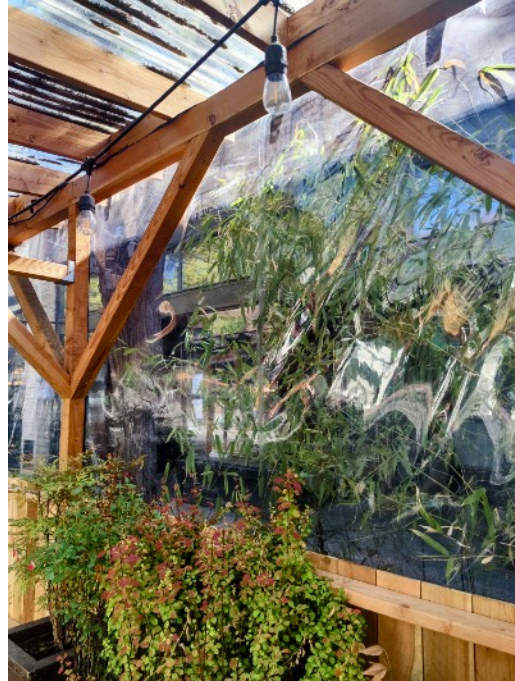
Photo 26: view of rain flaps from interior of patio
