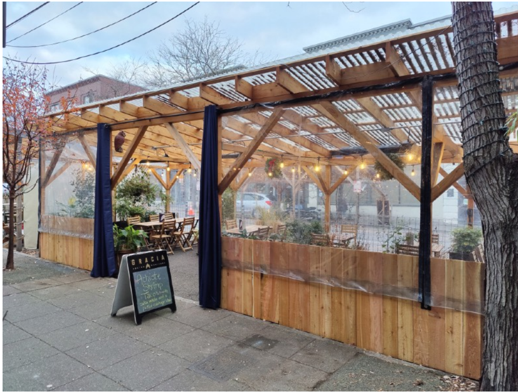
Photo 3: View from the south side looking north
