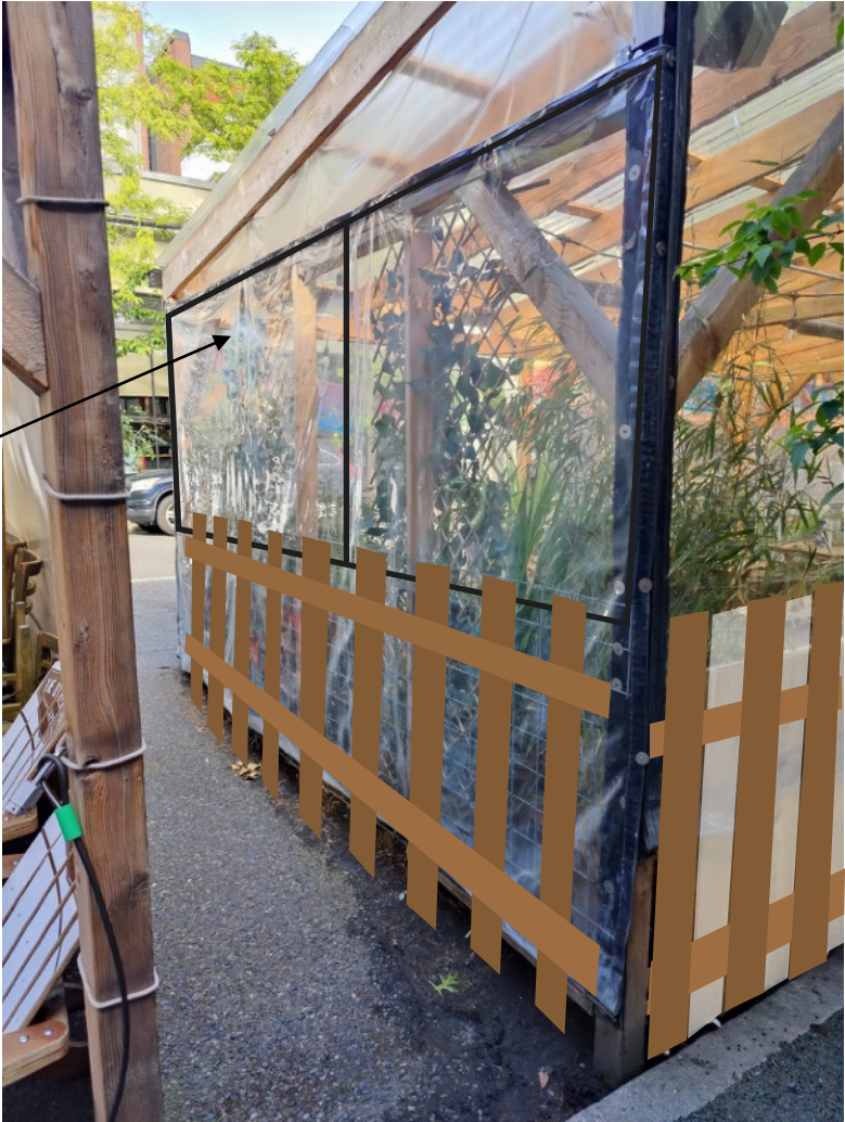
Photo 20: The photo to the right shows a mock up of replacing the metal fencing with the 42" tall Douglas Fir & Cedar plank fencing. Each plank is 5" wide with a 5" wide gap and features a toe rail for ADA accessibility.
