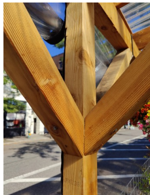
Photo 10: Detail of Douglas Fir joints detailing clear-coated weatherproofed natural wood grain
