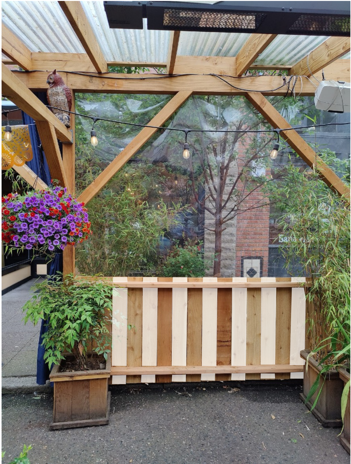
Photo 18: View from inside patio looking towards Gracia building. Fencing detail - the opaque lines represent the removed planks. Every other plank will be removed to comply with the SDOT ruling for 50% transparency in fencing.
