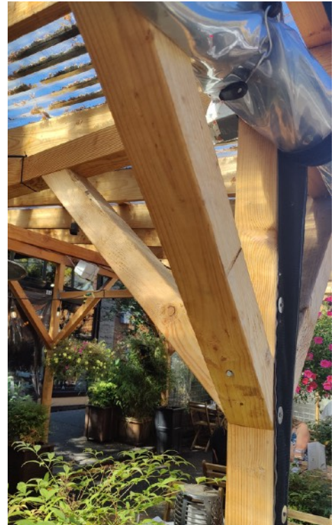
Photo 8: Detail of Douglas Fir joints
