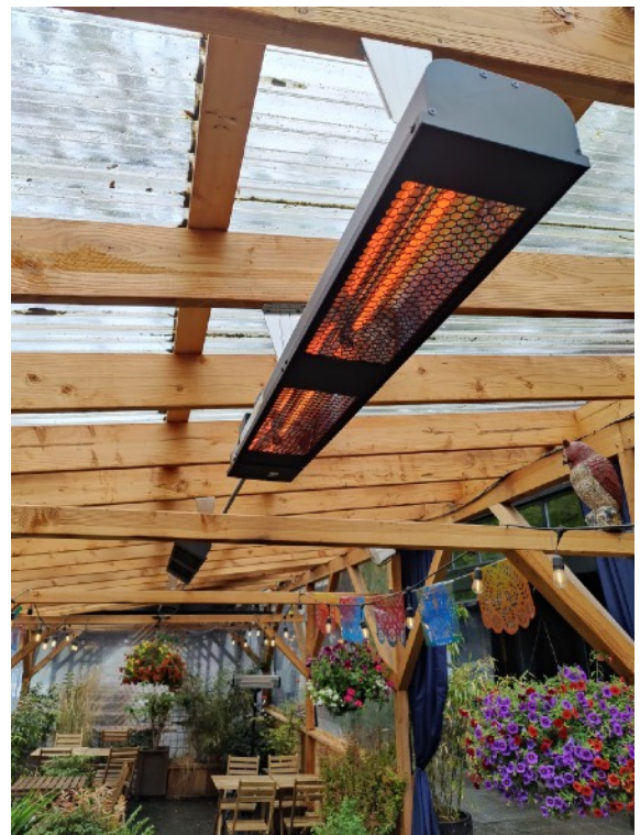
Photo 42: heater and roofing detail
