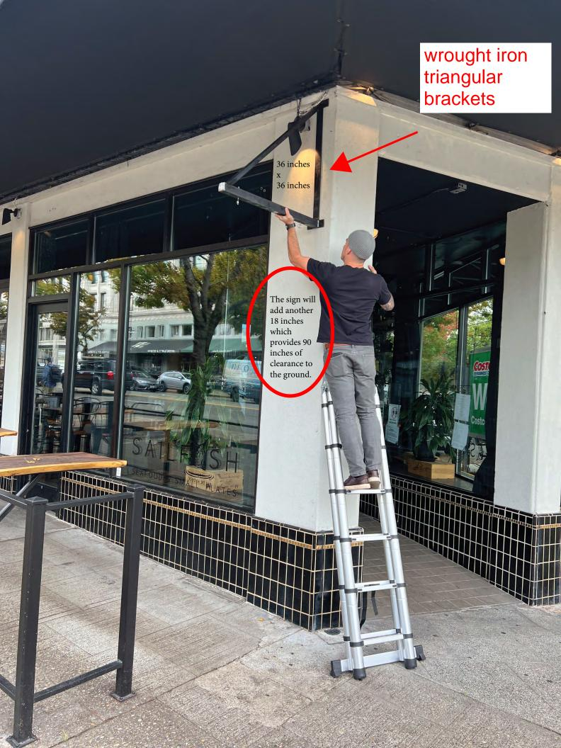
We will be using <u>4 inch SDS Galvanized Steel Lag Screws</u> to affix the signs to the building. In total there will be 8 holes from attaching the signs; 4 on each side of the building.
