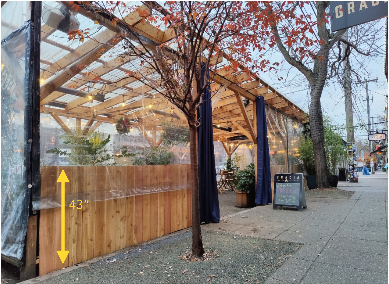
Photo 3: Patio shown from the north side. Note that every other wood plank will be removed and a toe rail will be added.
