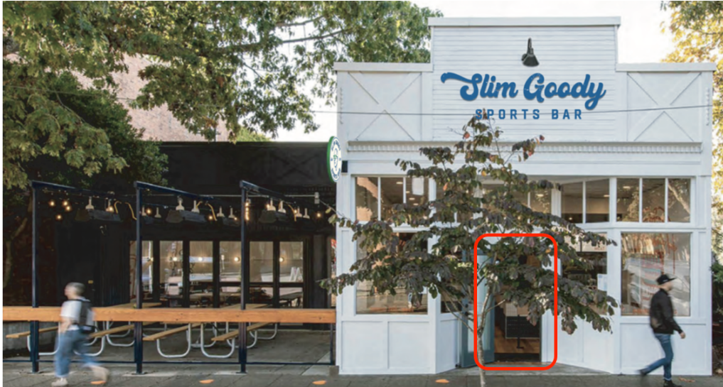
NOT PICTURED: STOREFRONT FACADE WAINSCOT REPAINTED SW9179 (SEE PAGE 06 FOR A PAINTED WAINSCOT IMAGE).
