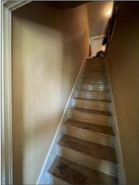
Missing Railing
