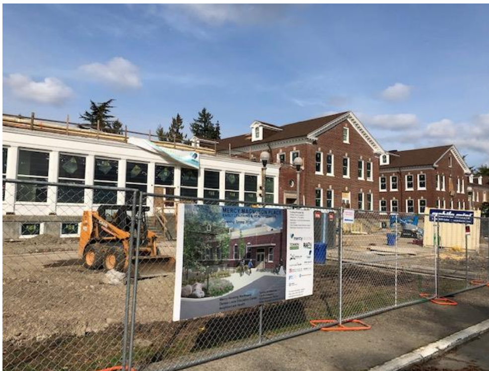
Building 9 Construction, Mercy Housing NW
