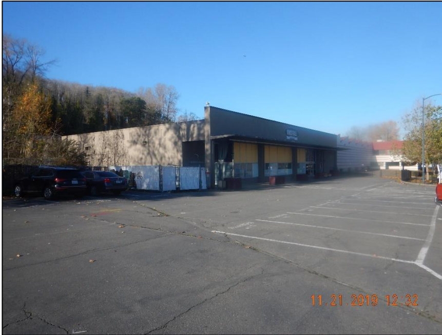
Plate 4: View of the former grocery store building in the south portion of the central parcel.
