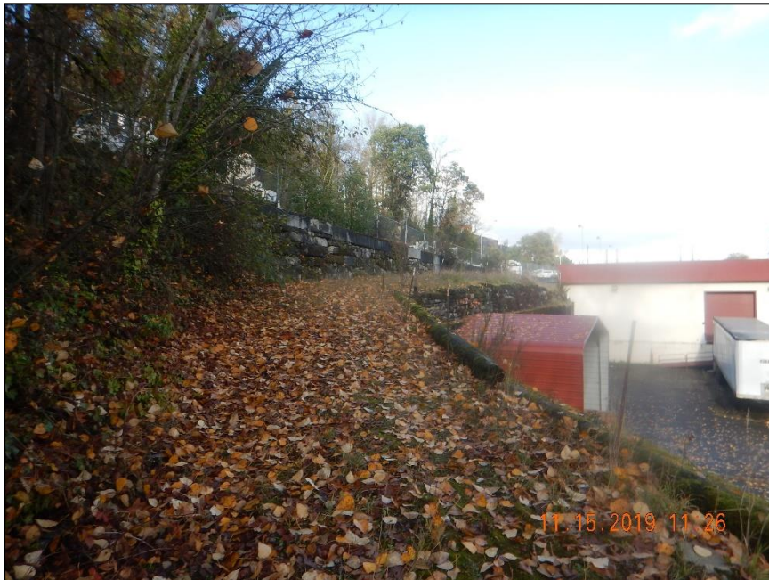
Plate 3: View of slope/access ramp on the west side of the UW Laundry site.
