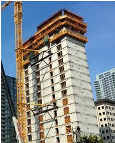
Figure 29. Reinforced concrete core building under construction.
