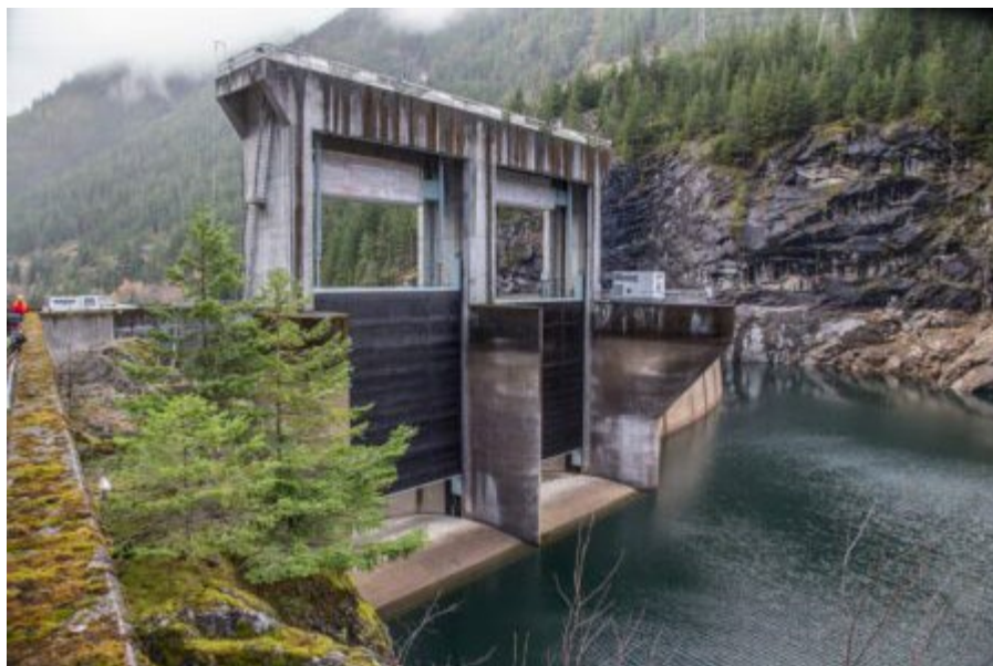
Gorge spillway gates
