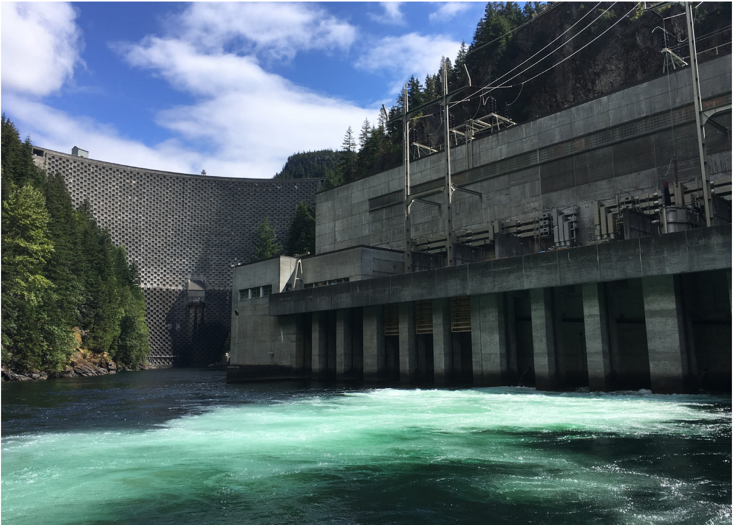
Ross Dam, the largest of the three hydroelectric dams that make up the Skagit Project.
