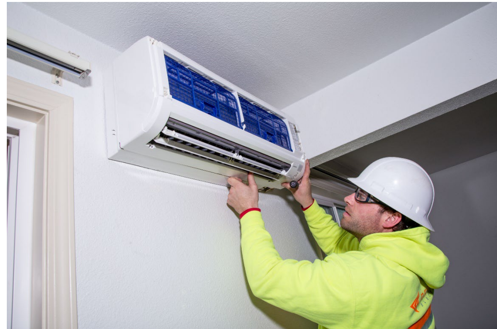
Energy-efficient heat pumps can heat and cool all in one unit. Image: Resource Media, Marcela Gara, Flickr Creative Commons.
