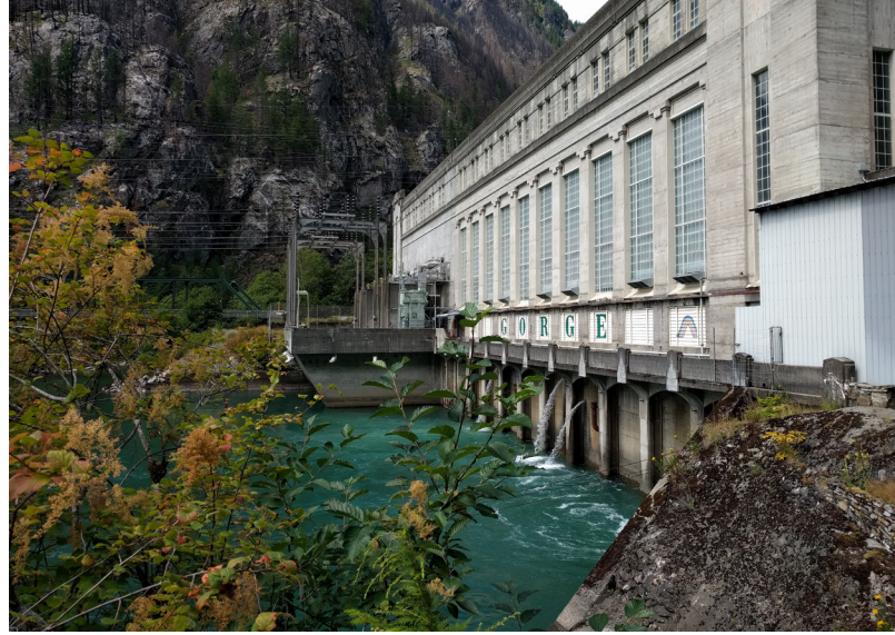
The Gorge Dam powerhouse.
