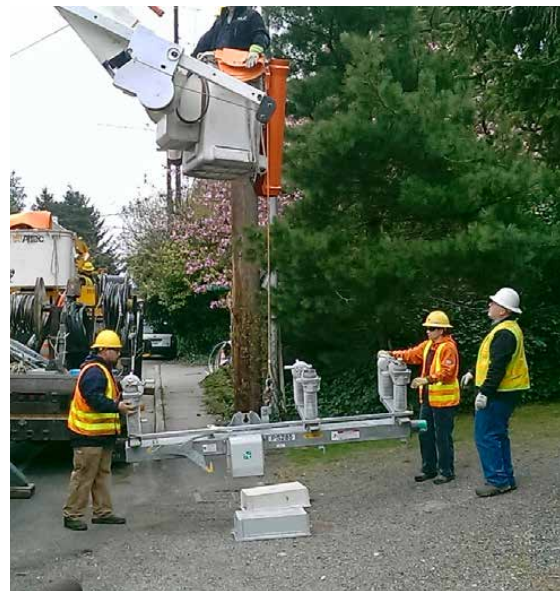
Lineworkers prepare to install an automated switch in Shoreline.
