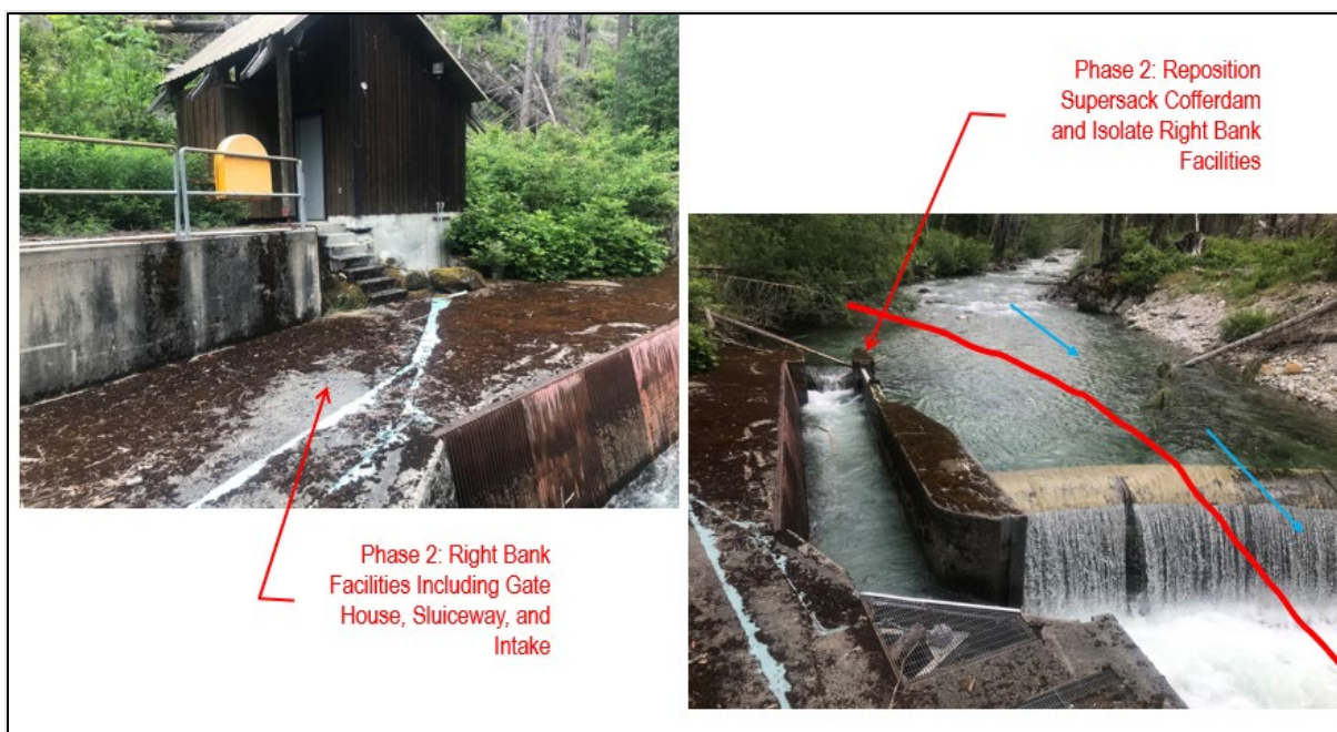
Figure 2.2-6. Right bank infrastructure to be removed during Phase 2.
