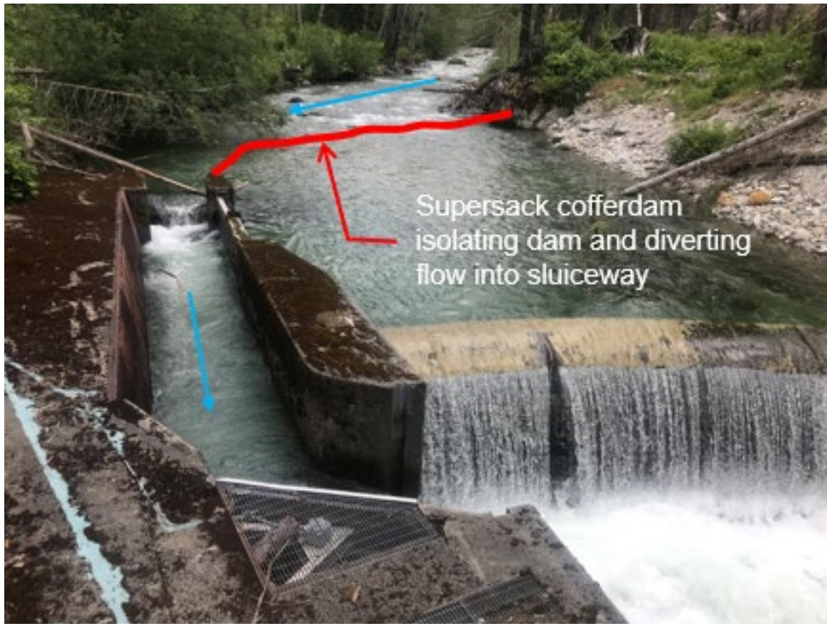
Figure 2.2-4. Photos depicting Phase 1 dam removal approach – divert creek into right bank sluiceway.
