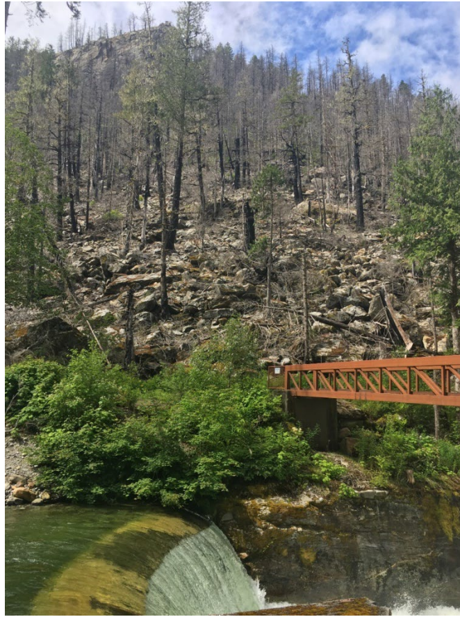
Figure 2.2-8. Newhalem Creek diversion dam pedestrian bridge, showing left bank abutment downstream of the dam.
