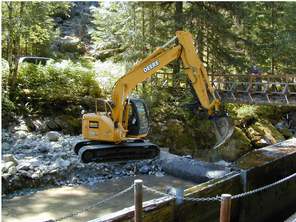
Figure 4.1-1. Annual excavation and downstream redeposition of accumulated gravels and cobbles upstream of the Newhalem Creek diversion dam (2005).
