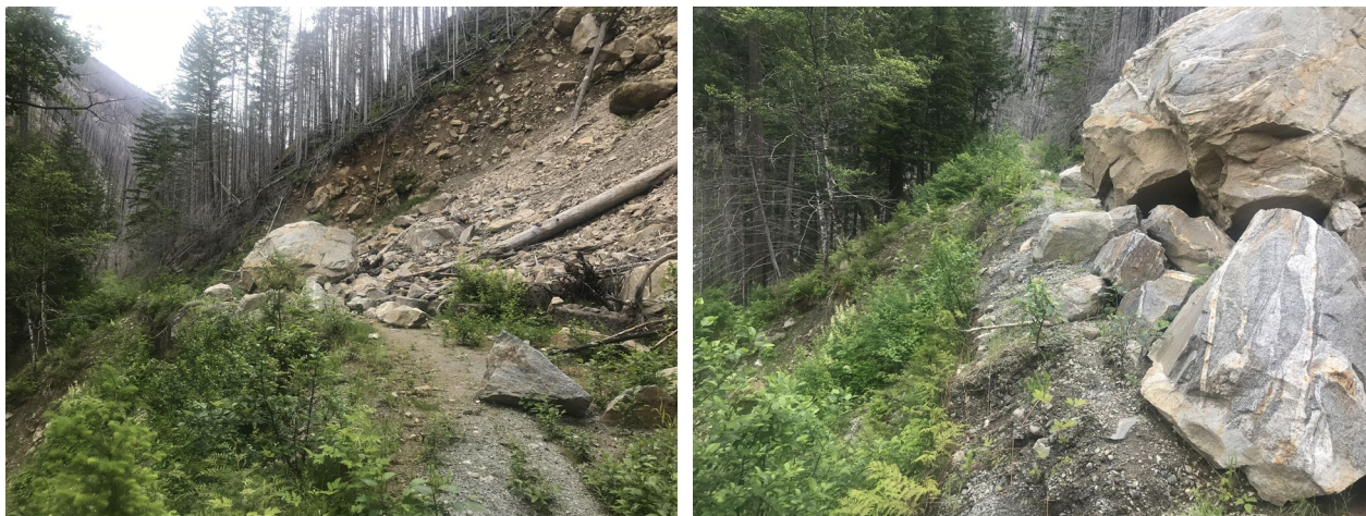
Figure 2.2-1. Photos of Dam Access Road showing landslide and embankment instability.
