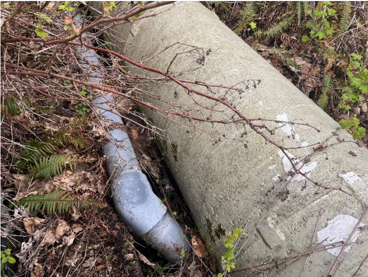
Figure 5. Six-inch diameter PVC pipe adjacent to the penstock.
