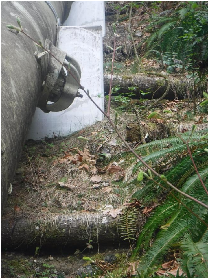
Figure 10. Untreated logs and concrete saddles on the steep slope just above the Powerhouse.
