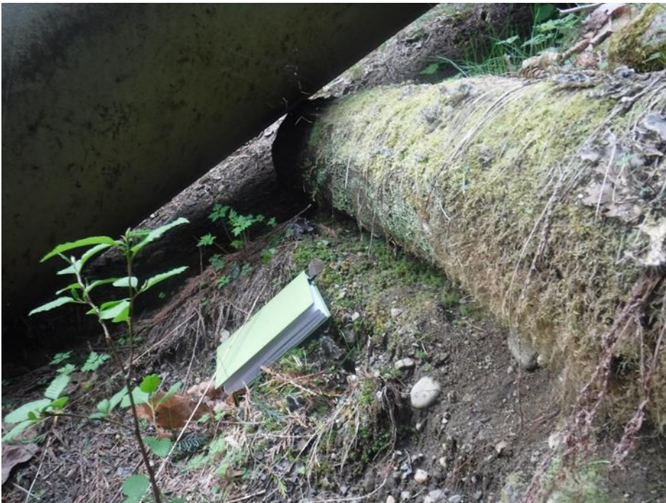
Figure 8. Drainage pipe near the steep slope adjacent to where the penstock exits the tunnel, minimal water flow is poorly dispersed.
