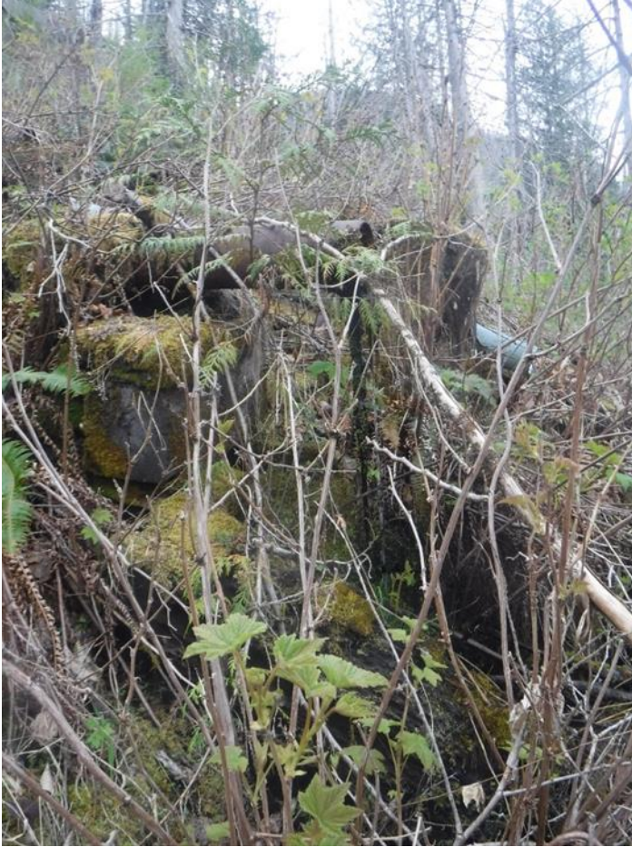
Figure 8. Drainage pipe near the steep slope adjacent to where the penstock exits the tunnel, minimal water flow is poorly dispersed.
