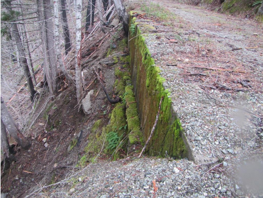
Figure 13. Cement retaining wall associated with the access road to the headworks.
