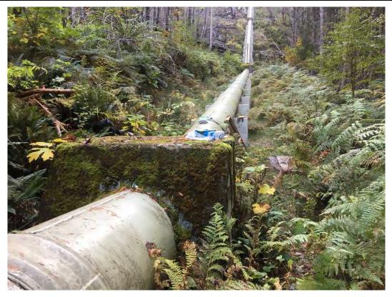
Photograph 7. Thrust Block III in foreground; view to south.
