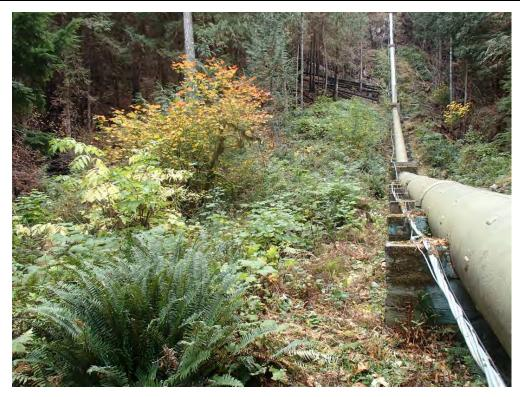
Photograph 3. Before saddle replacement: former creosote-treated wood saddles between Thrust Block II and III; view to south; October 2015.
