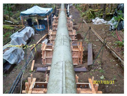
Photograph 4. During saddle replacement: soil excavation during saddle replacement; view to the south; March 2017.
