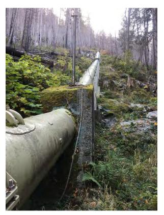
Photograph 10. Thrust Block IV with slight surface flow on bedrock adjacent to saddles.
