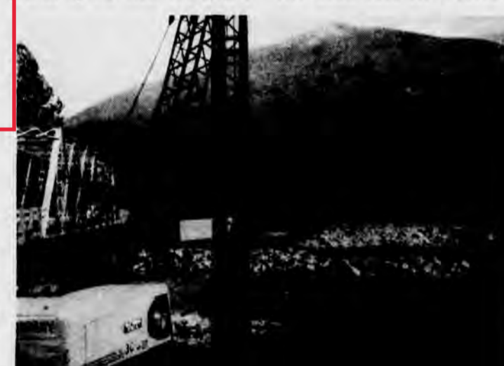
CASCADE BRIDGE STARTED The contractor is now on the job at Cascade River, above Marblemount, putting in piers for a new span to replace the old plank bridge (left) which has served for many years.
