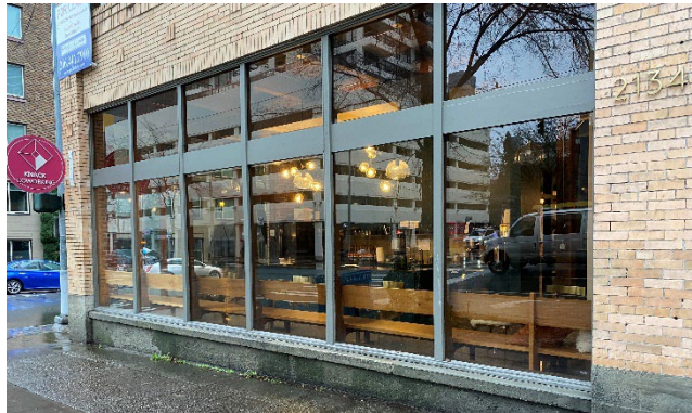
Figures 6-7-8: Exploring other strategies for marketing will provide an opportunity for the business in top left photo to remove ads from storefront windows, opening views to the street that can attract customers and deter criminal and unwanted activity. Top right and bottom photos depict businesses with open views, adding vibrancy and increasing informal guardianship on the street.
