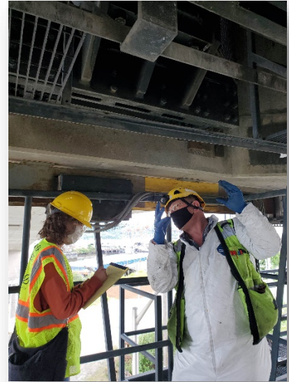
OCA Auditor and SDOT Inspector at the Spokane Street Bridge, July 2020.
